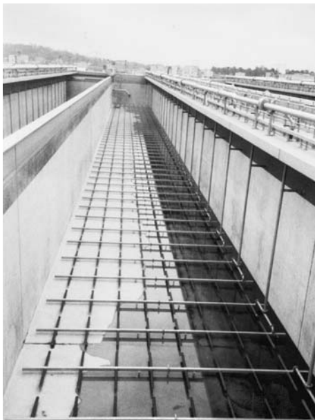
Fig. 5.10 Porous ceramic tubes in deep tank aeration, second zone of a longitudinal tank at WWTP Waßmannsdorf, near Berlin (Schuchardt et al. 2002).
