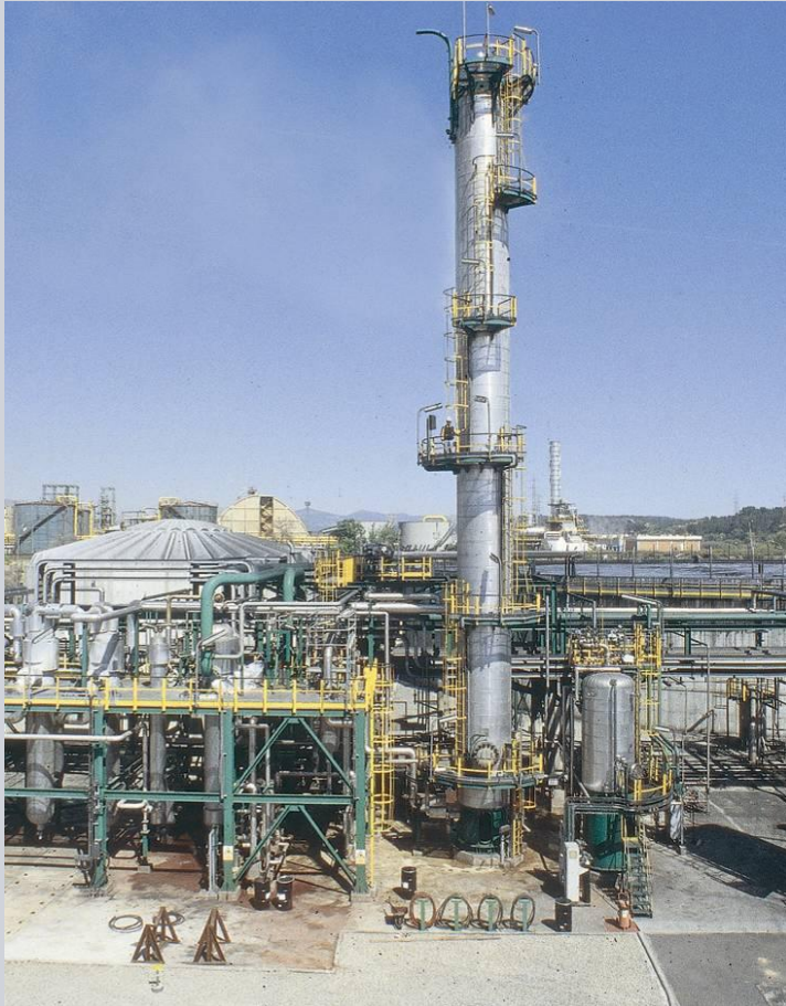
Repsol, Tarragona, Spain
