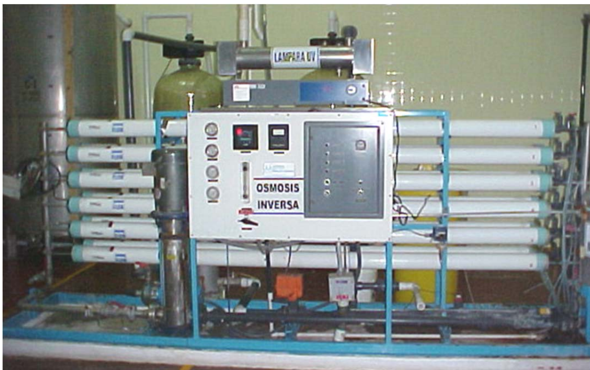
Packaged skid with instrumentation, UV, and softening unit.
