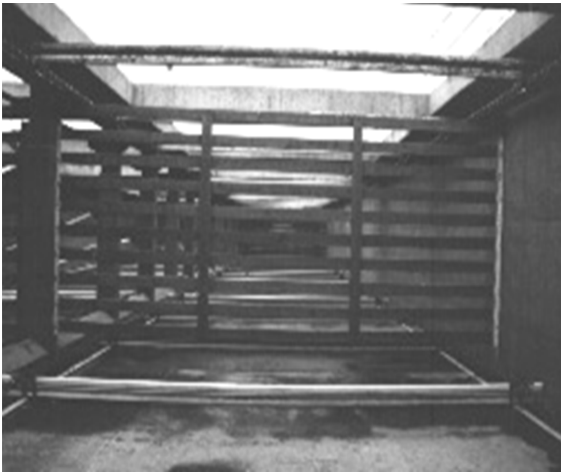
Rectangular basin flights and chains.
