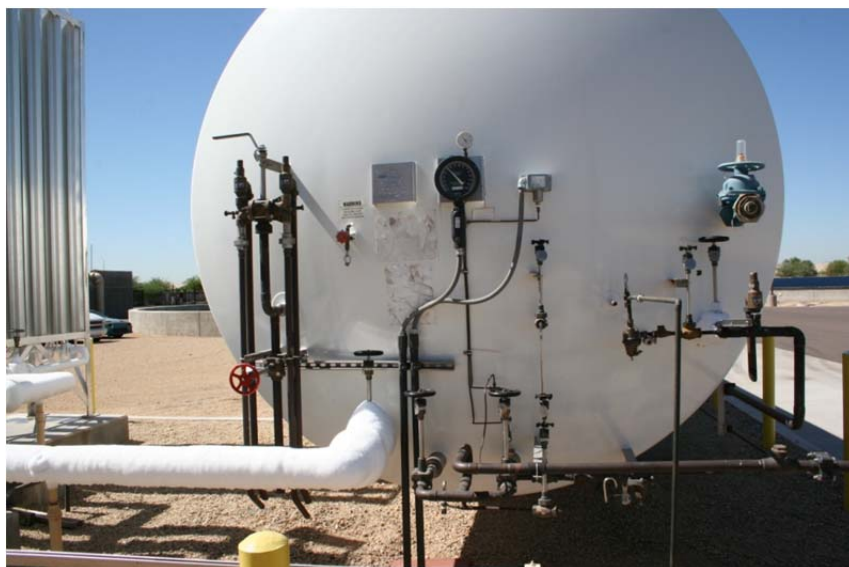
An onsite Oxygen tank is necessary to generate O_3
