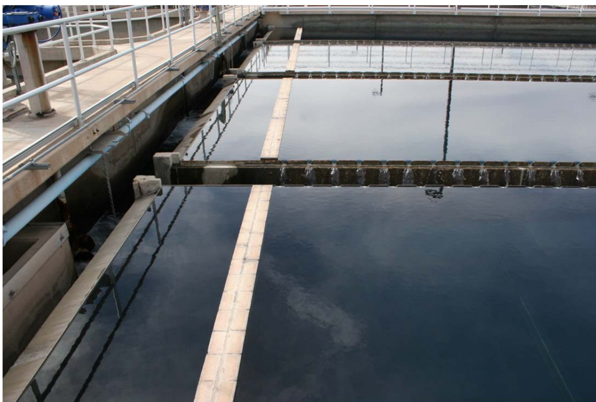
Rectangular basin flights and chains.
