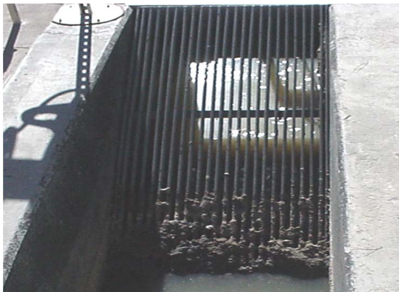
Mechanical bar screen
