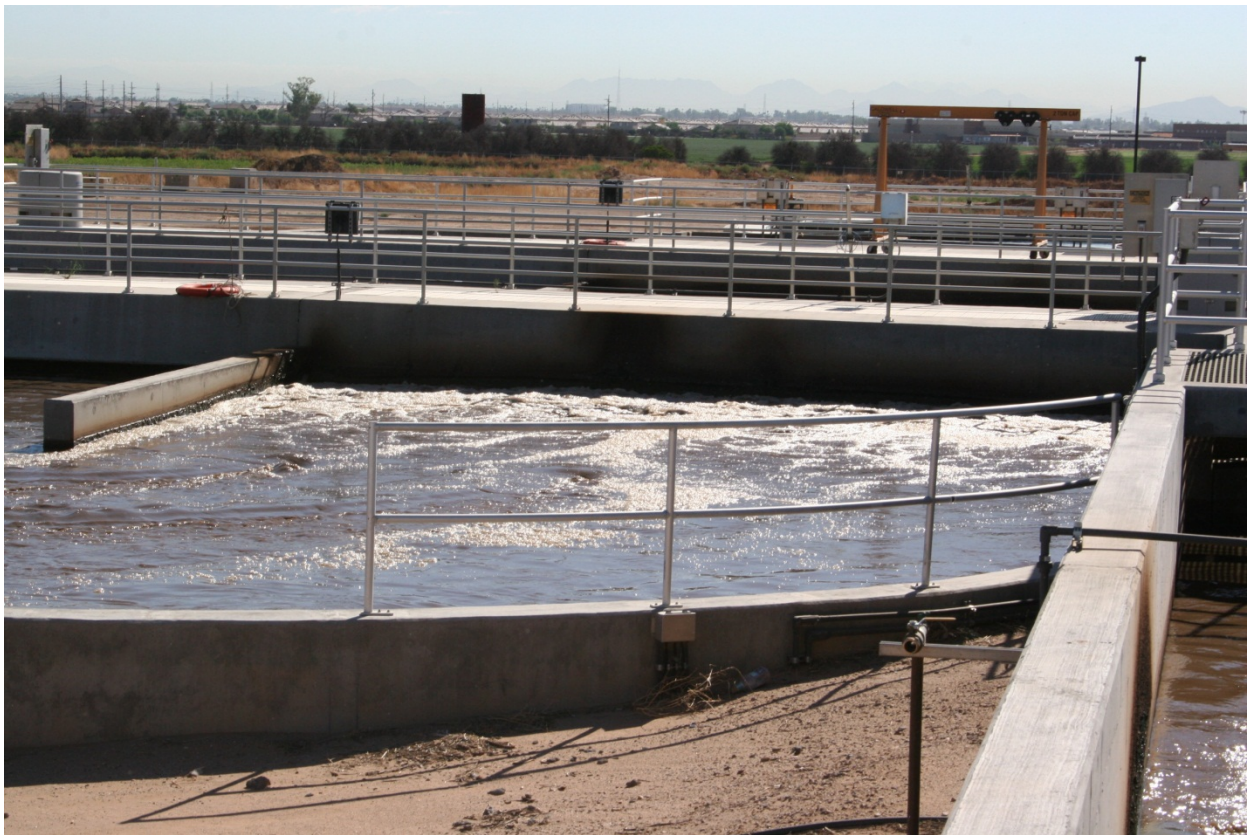
Oxidation ditches are used for nutrient removal.
