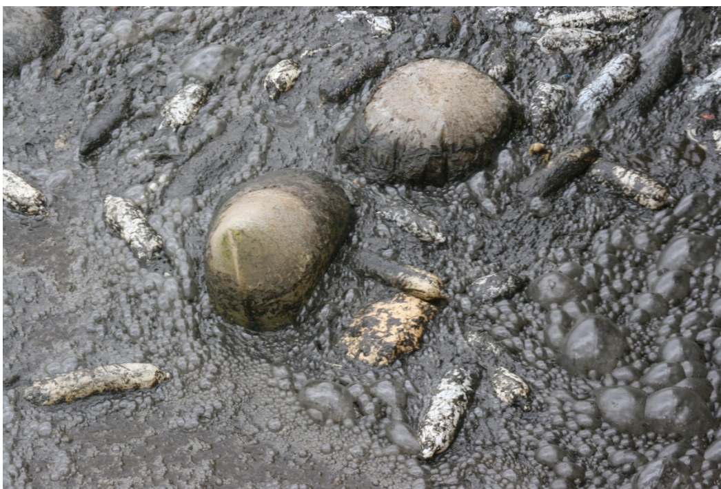
Floating scum in primary clarifier.
