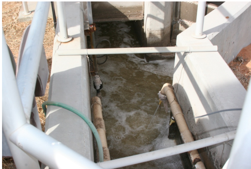
Aeration is often used to refresh the wastewater flow at the influent channel.
