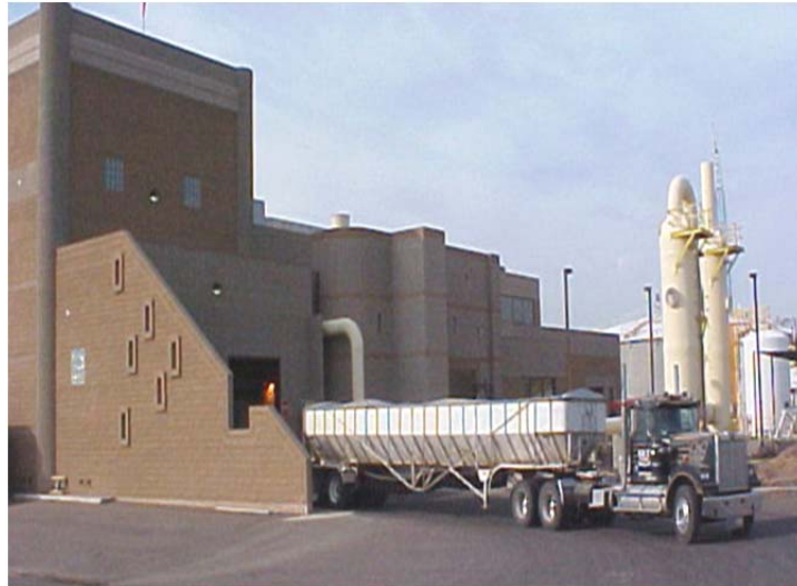
Large solids treatment facility
