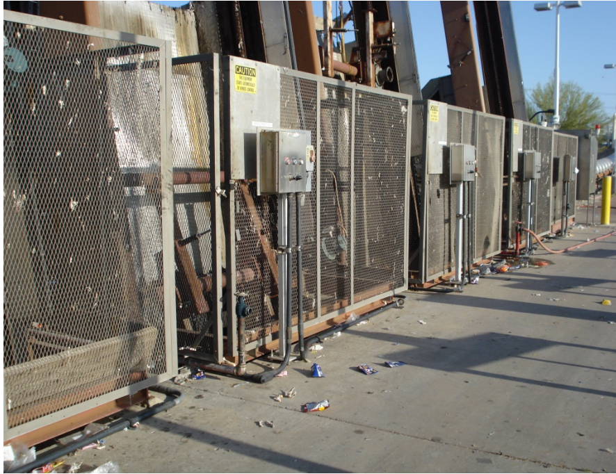
Mechanical Bar Screens. Operators are necessary to pick up trash that is blown off the rakes.
