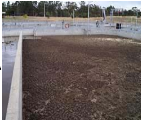
Figure 3. Dry Microthrix parvicella foam trapped in an anoxic zone of a BNR plant aeration basin.
