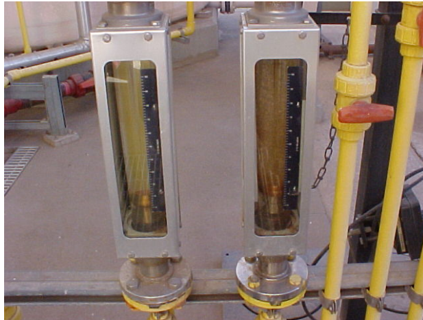
Chlorine measurement devices or Rotometers.
