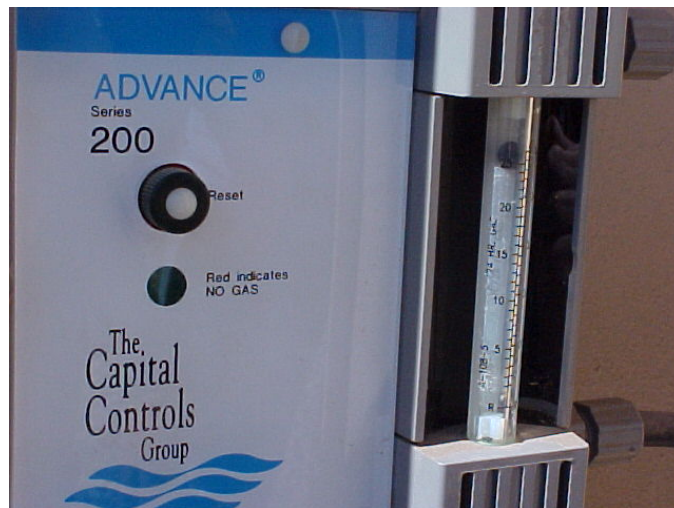
Chlorine measurement devices or Rotometers.
