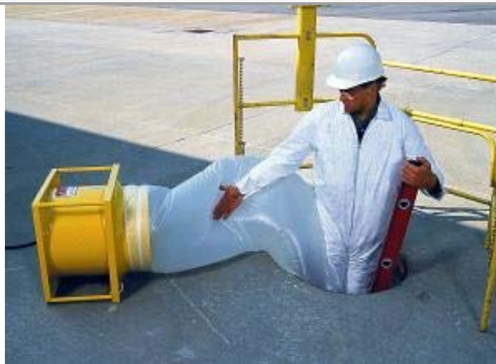
Forced air ventilation with a disposable air shaft. Typical Display of the TMX412
