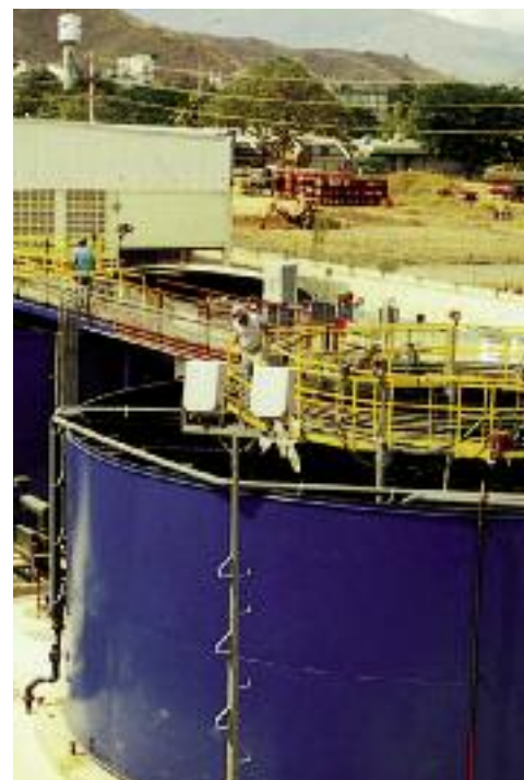
Our package plants for biological treatment can economically handle clarification, aeration and digestion in a single modular unit.
