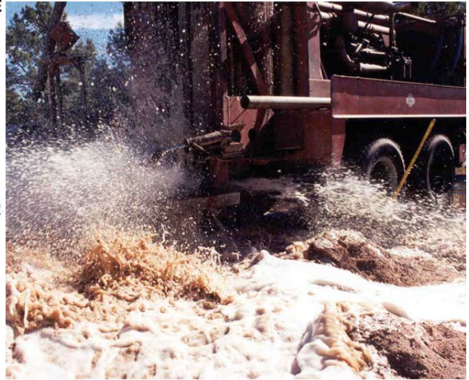
Surge of air developing a Well.
