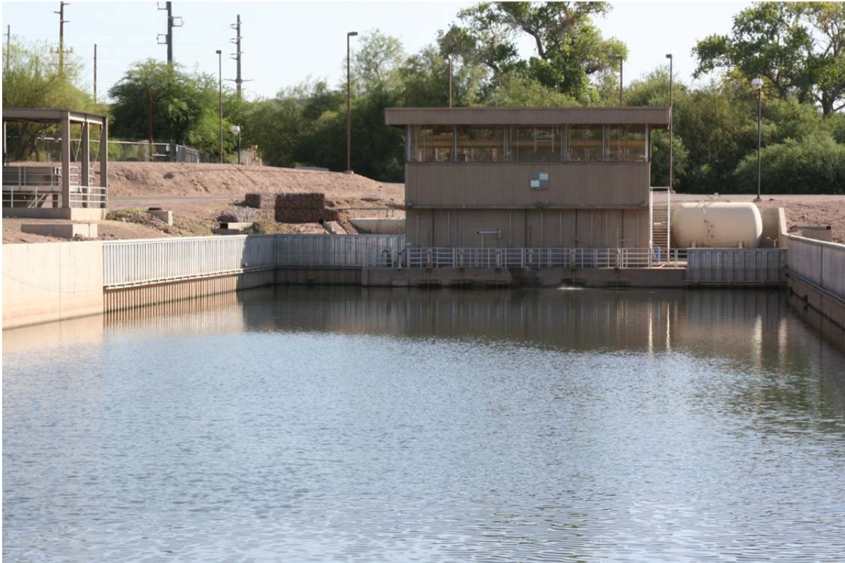
Raw Water Intake
