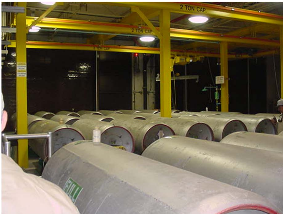
1-ton chlorine gas containers.
