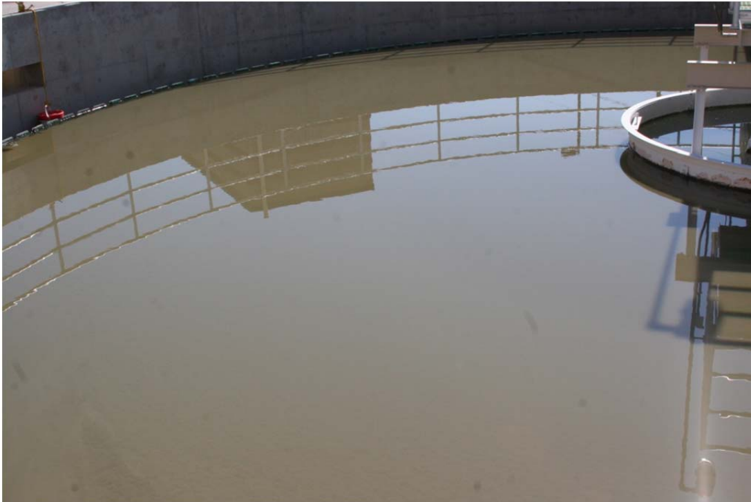
Top- Pre-sedimentation basin
