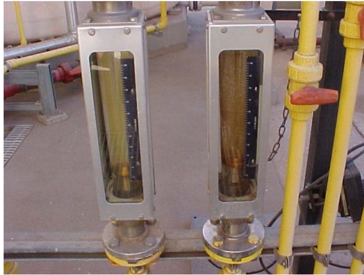
Chlorine measurement devices or Rotameters.
