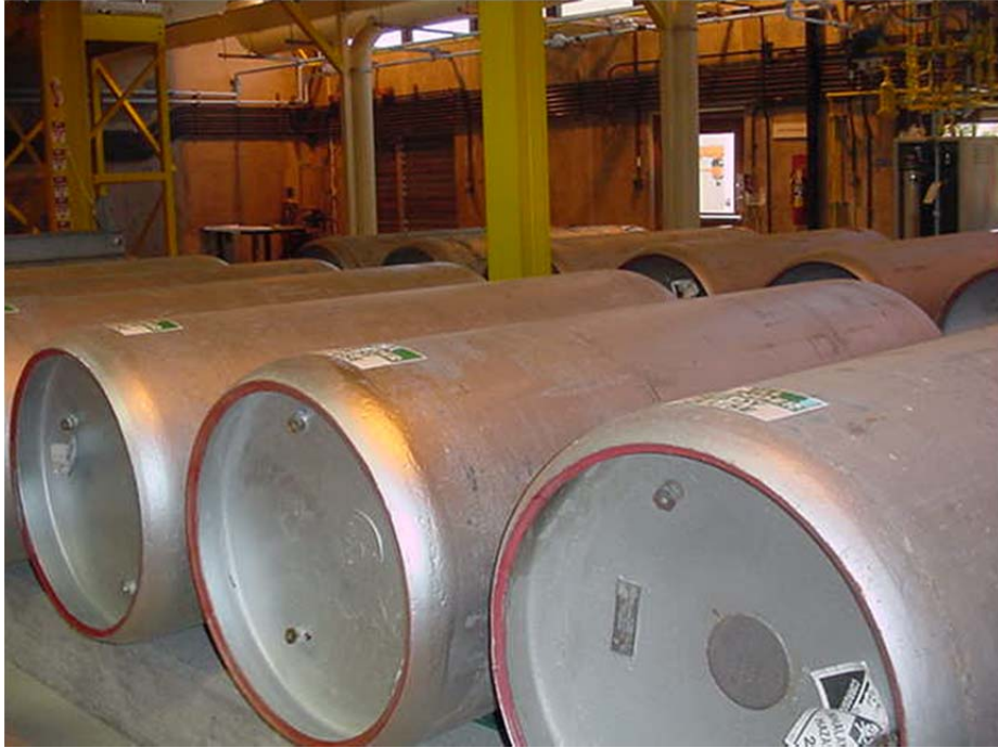
1-ton chlorine containers, rear side of container.
