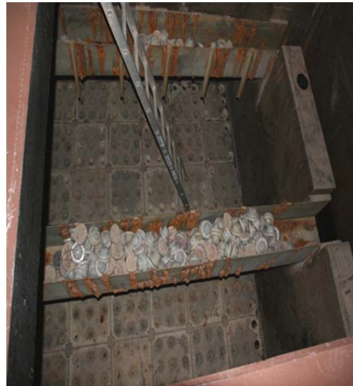
The photograph on the right shows a filter support bed under construction.
