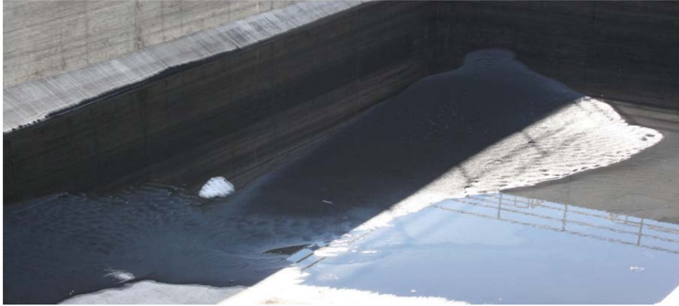
A photograph of a backwash basin that has media caked on the bottom.
