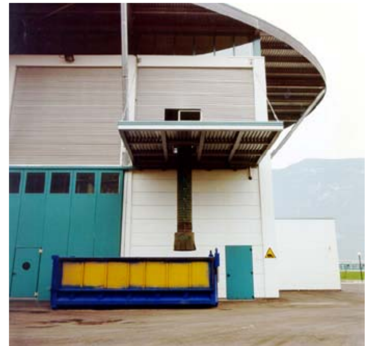
Dried product discharge telescopic unloader
