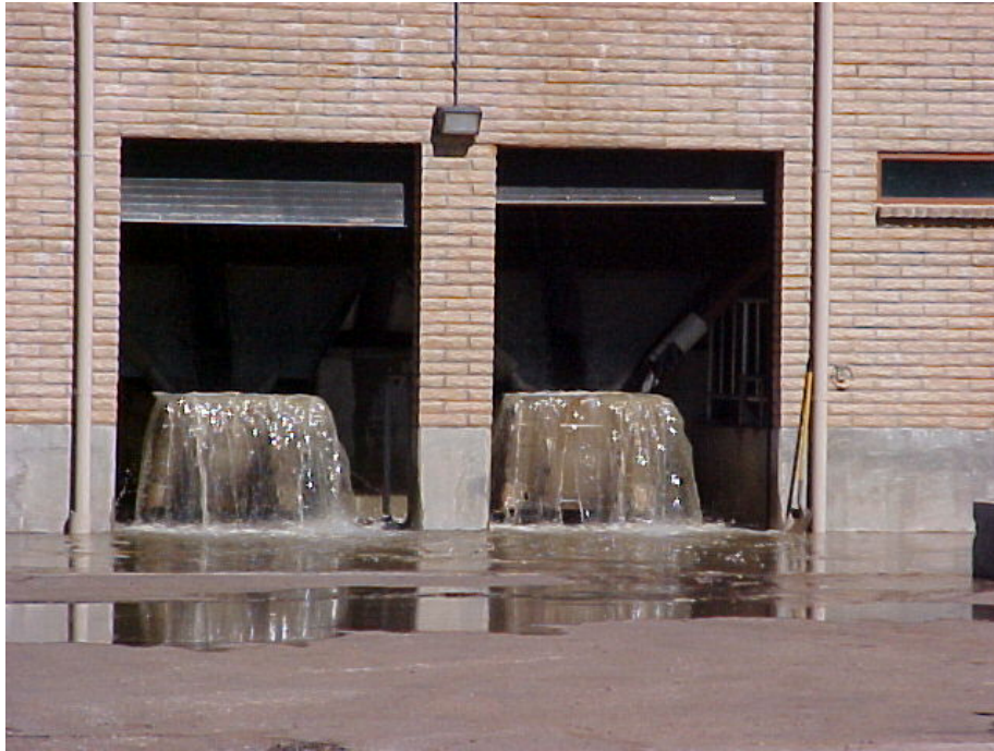
Effects of a clogged bar screen causing Headworks to flood. This mess was caused by grease clogging up and happens frequently at this WWT facility. It is time to hammer the violator of the grease problem.
