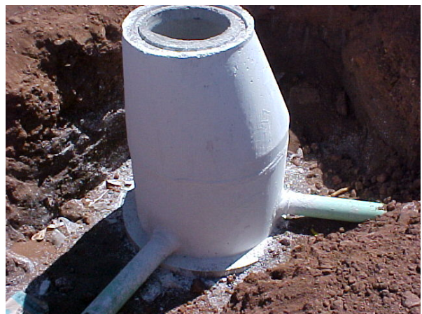
Newly finished Manhole and Laterals.
