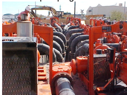
Pumps at a temporary sewer manhole by-pass.
