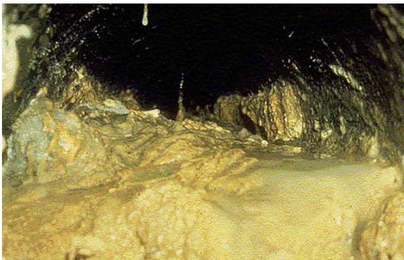
Grease build-up inside a sewer causing interference with flow.
