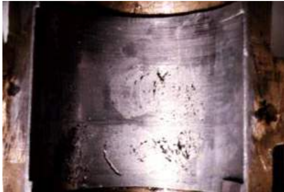
(a) Fatigue Damage in its Early Stages
