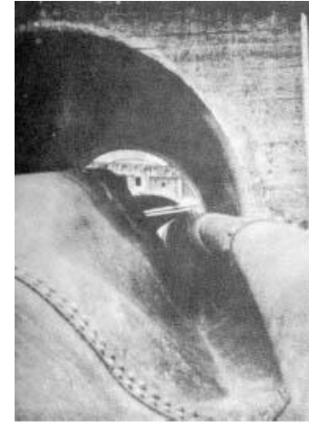
Pipe damage in power station Okigawa
