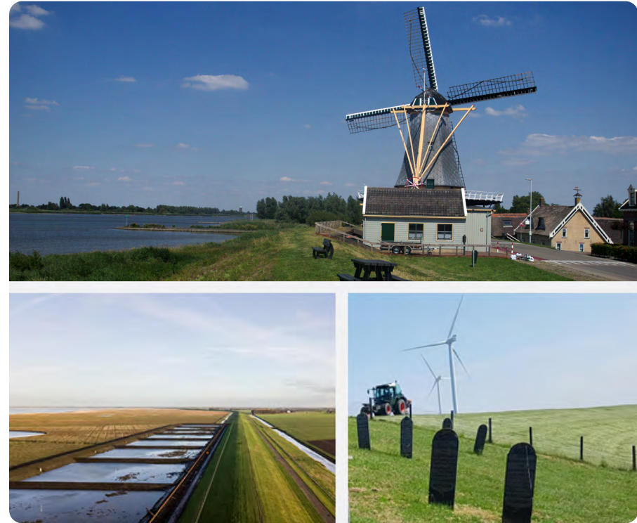
Figure 2: Range of functions that can be encountered on/near a flood defence including housing on a riverine dike ( top photo ), vegetated foreshores in coastal areas with adapted design for the extraction of deposited clay ( bottom-left ) and more (unusual) objects that can be found ( bottom-right ). Photos respectively obtained from Flickr (by Grotevriendelijkereus , CC BY-NC-SA 2.0 ), Regional Water Authority Hunze en Aa's and Richard Marijnissen.
