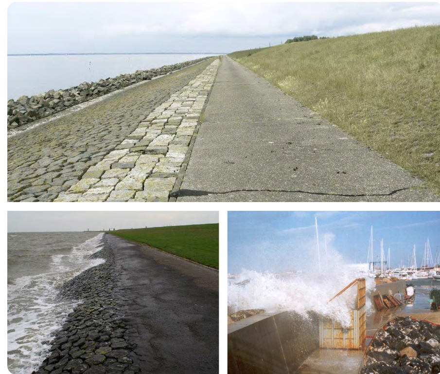
Figure 2: Top: Various types of roughness elements and a berm applied at a dike. Source: EurOtop (2018, p.103) . Bottom: Wave run-up and overtopping at dikes in the Netherlands (left) and embankments in Italy. Source: EurOtop (2018, p.103 and p. 51) .
