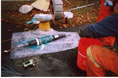
.Sleeve Grouting with Copper Sulfate -12
