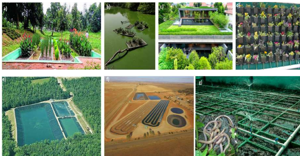
Figure 4.2.1: Nature-based solutions a) constructed wetlands, b) floating treatment wetlands, c) Green roofs, d) living walls, e) waste stabilization ponds, f) high-rate algal ponds, and g) vermifiltration
