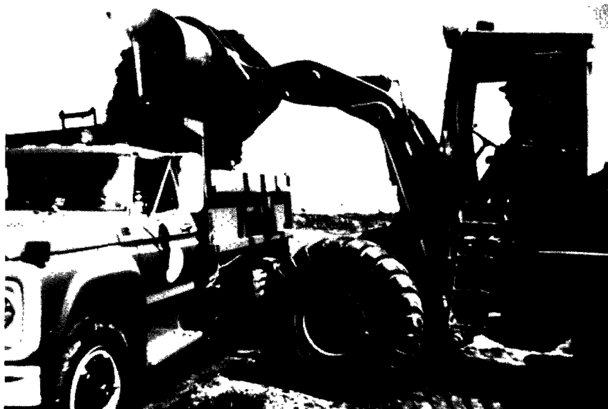
FIGURE 11-14 UNLOADING SLUDGE INTO WIDE TRENCHES WAUKEGAN, IL
