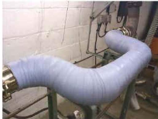
(b) White Insulation on Top
