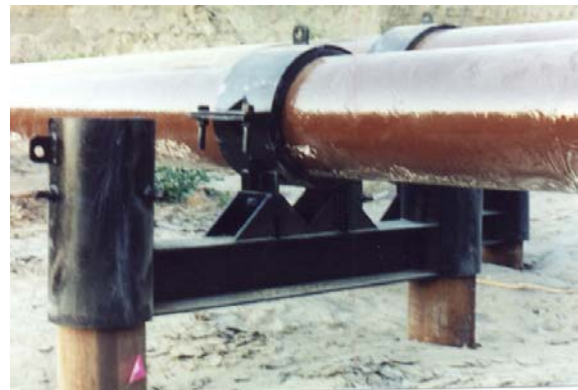
Figure 2.12: Clamped Support
