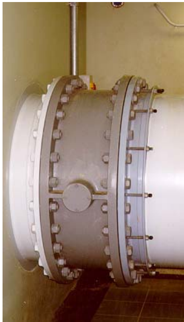
(b) Two Designs of Pipe-to-flange Adapters Fitted
