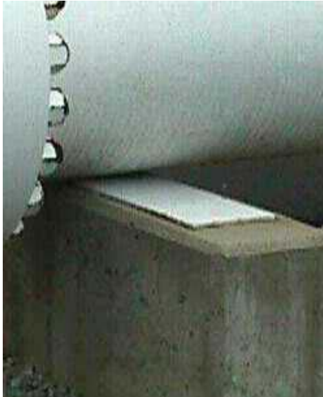
Figure 2.11: Simple Concrete Support Block
