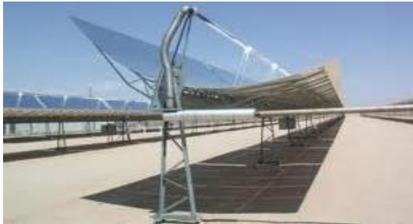
Fig. 11: Parabolic trough solar collector
