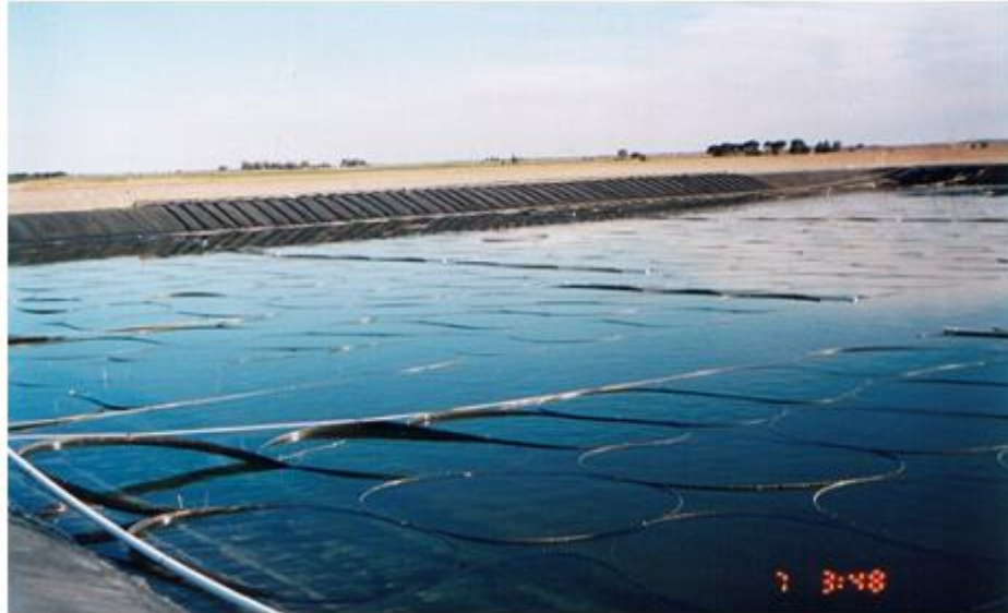
Fig. 2: Demonstration solar Pond at Pyramid Hill in Northern Victoria
