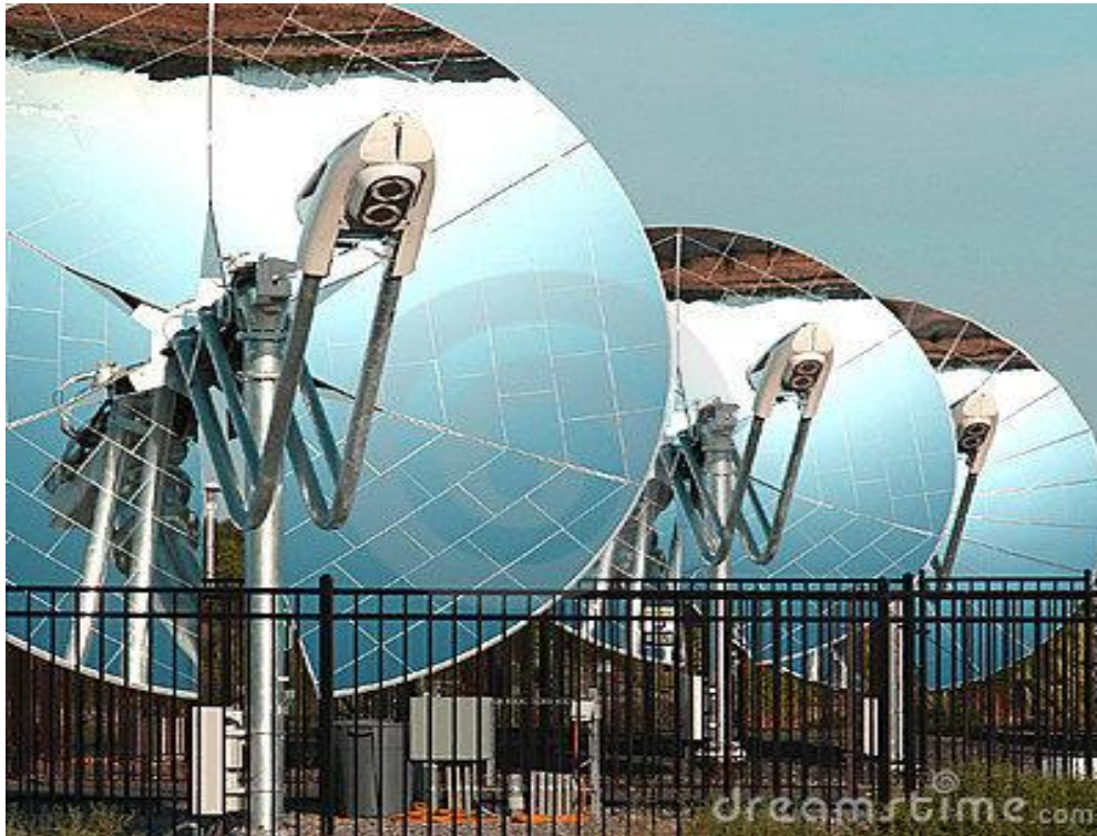
Fig. 15: Parabolic dishes solar collectors with their trackings
