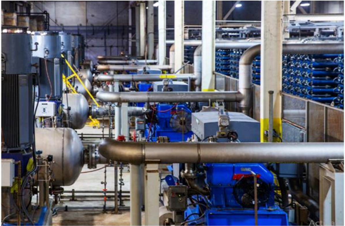
High pressure pumping system at the Tampa Bay Seawater Desalination Plant
