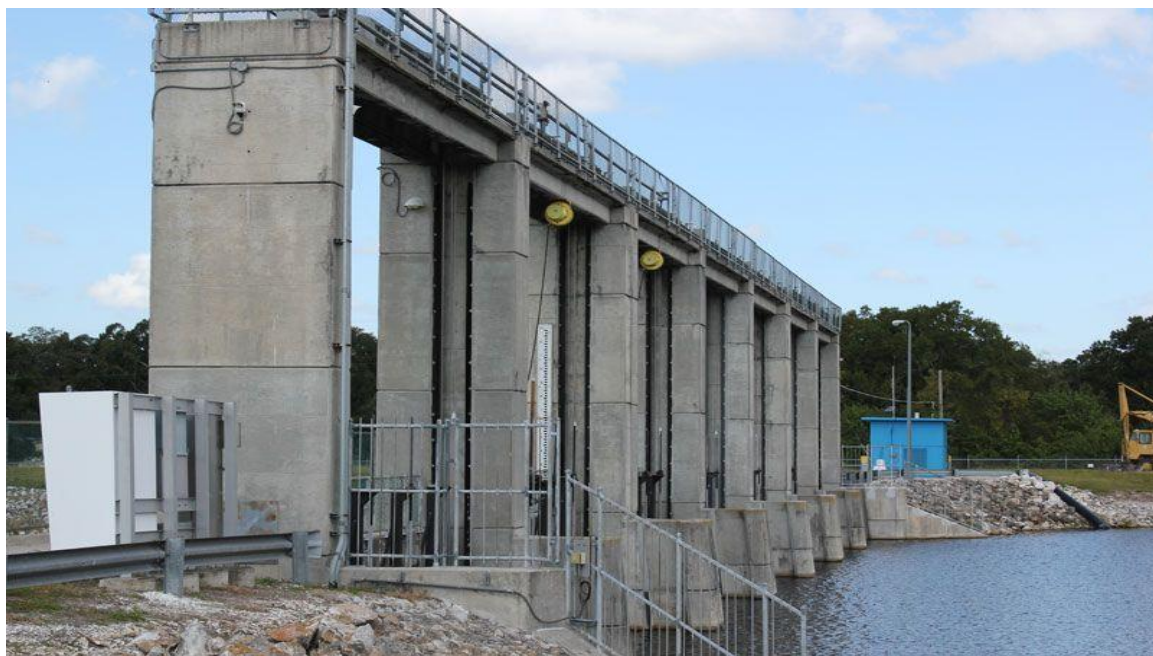
Tampa Bypass Canal Intake Structure.
