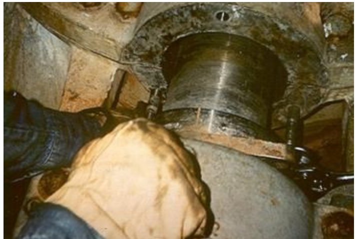
Typical shaft finish after removal of gland packing
