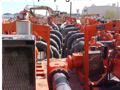
Pumps at a temporary sewer manhole by-pass.
