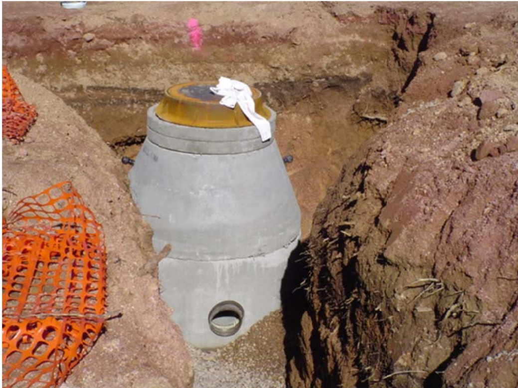
Top photograph, new manhole. Bottom, a repaired sewer main after being damaged by the water distribution department using a backhoe without locates.
