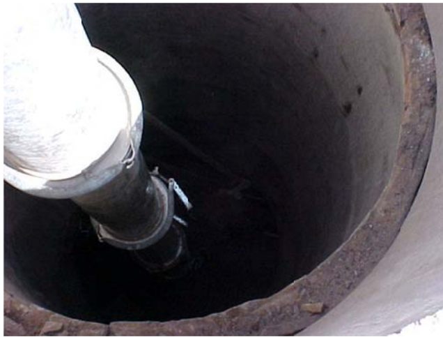
Looking down inside the manhole.
