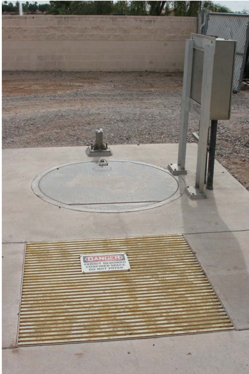
Lift Station used to convey sewer or collections to a higher location in the system.
