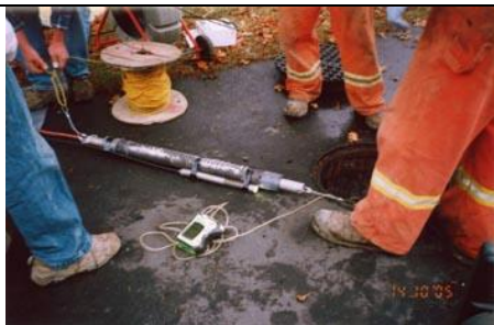
The Installation Sewer Plug -8
