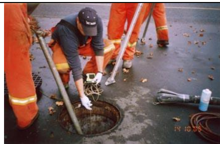
Testing the gas level -7
