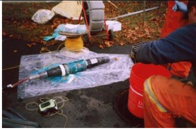
.Sleeve Grouting with Copper Sulfate -12
