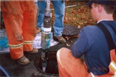
..Lowering the Sleeve to the Manhole -14
