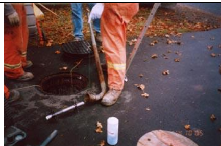
See Snake CCTV preparation -9
