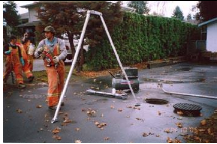
.Installation Crew in action -3
