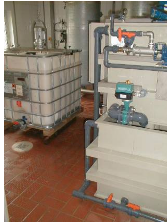
Polymer Preparation Station
