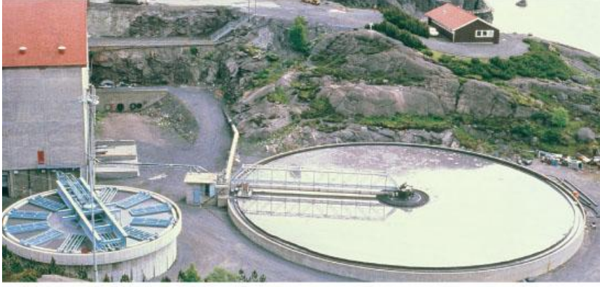
Installation of a Svedala LTC Combi lamella clarifier next to a conventional round thickener with approximately the same clarification area.
