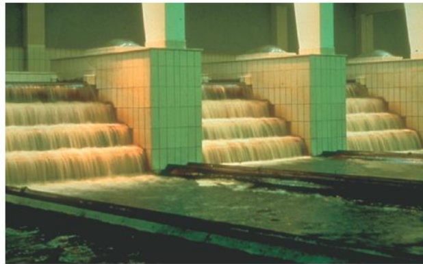
Figure 7 - Treatment of slightly anaerobic groundwater
