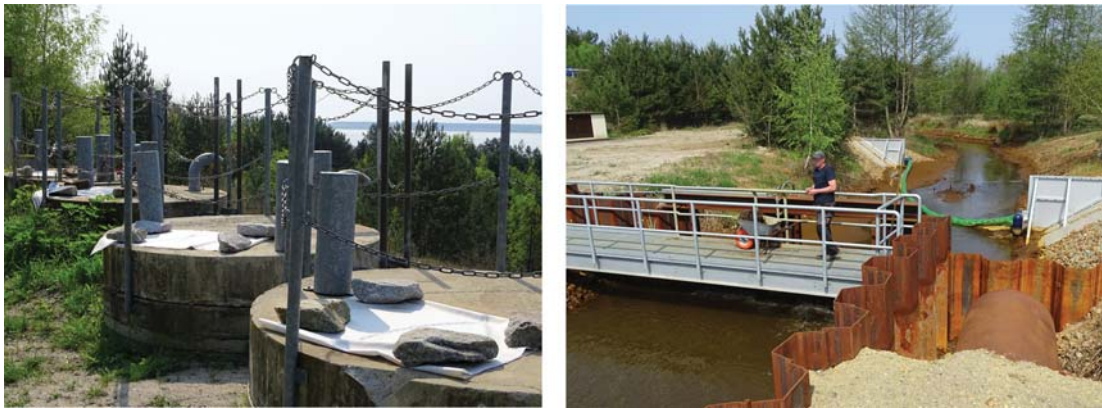
Figure 7.9 Rehabilitation of lignite mines: the case of Lusatia (Germany). Left: groundwater management, right: flooding water channel to fill an open cast mine chain. (Photographs: Petra Schneider )
