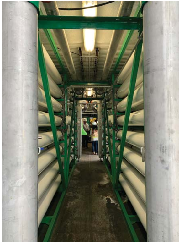
Figure 25.2 Reverse osmosis filtration system is used to treat foundation drainage for reuse at Energy Center San Francisco. Similar smaller systems are used to treat brewery process water for reuse at breweries. (Credit: San Francisco Public Utilities Commission)
