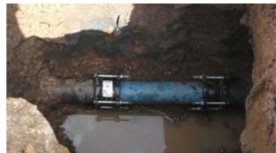
Figure 38 Typical repair couplings and installation (Sources: Mueller Water Products Inc. (1), Plasson (2), D Pearson (3)).
