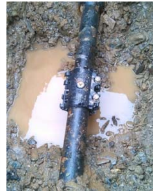
Figure 37 Typical repair clamps and installation (Sources: Plasson (1, 2), K Atkinson (3)).
