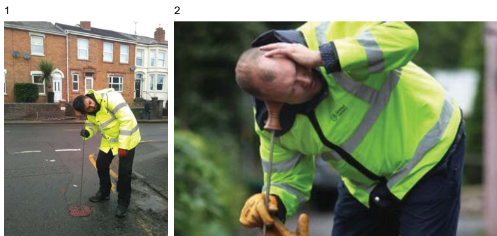
Figure 30 Photographs showing use of manual listening stick (Sources: K Atkinson (1), United Utilities (2)).
