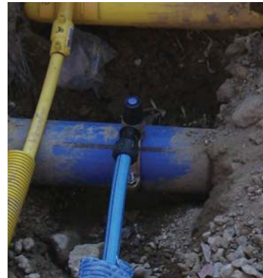
Figure 12 Typical tapping tees and installation (Sources: Aliaxis UK (1), Mueller Water Products Inc. (2), J Parker(3)).
