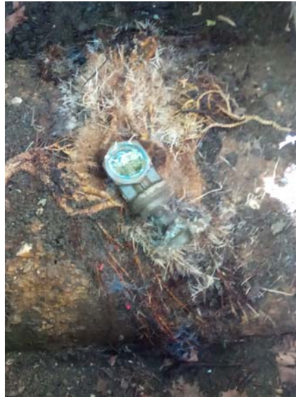
2 Installation on pipe
