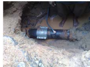
Figure 13 Typical ferrule and installation (Sources: Mueller Water products Inc. (1), K Atkinson (2)).
