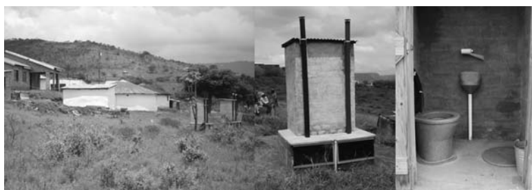
Figure 33.1 Images from left to right: peri-urban settlement with two UDD toilets on the right; a typical double-vault urine diversion dry toilet; inside view. © Duncan Mara
