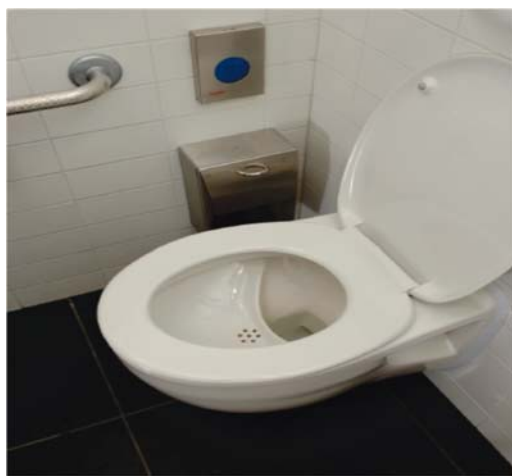
Figure 6.11 Roediger NoMix toilet. Roediger Vacuum ( www.roevac.com ) (Reprinted from Larsen T. A., Alder A. C., Eggen R. I., Maurer A. and Lienert J. Source separation: will we see a paradigm shift in wastewater handling? Environmental Science & Technology , 43(16), 6121–6125, with permission from American Chemical Society).
