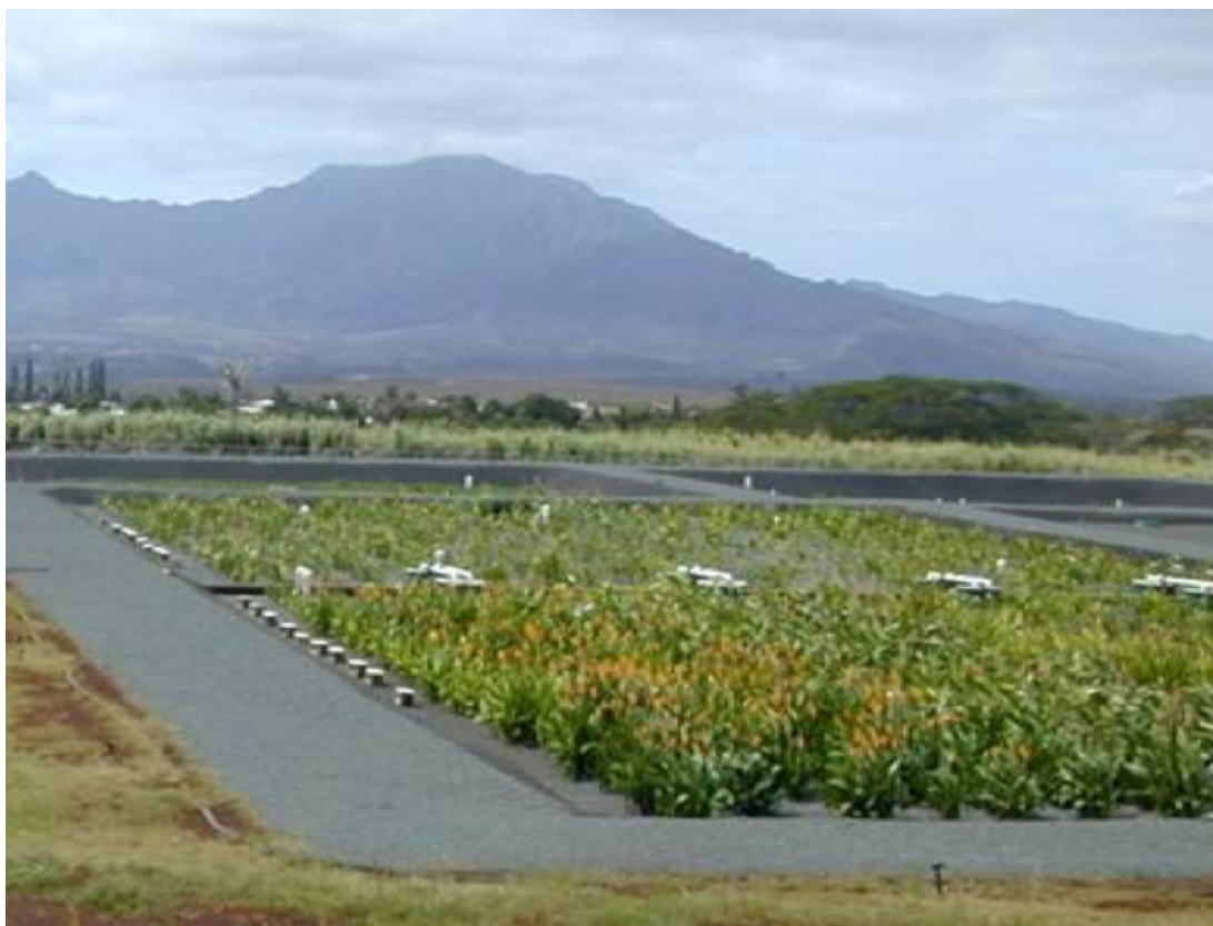
Figure 1: Two-cell reciprocating TW for treating municipal wastewater, Wahiawa, Oahu, Hawaii. Each cell was 27.4 \text{ m} \times 27.4 \text{ m} \times 1.2 \text{ m} deep. Notice four sets of opposing pump wells for timed fill-and-drain reciprocating operations. Treatment cells were planted with several varieties of tropical Heliconia spp. for aesthetics and as a proposed cut flower demonstration.
