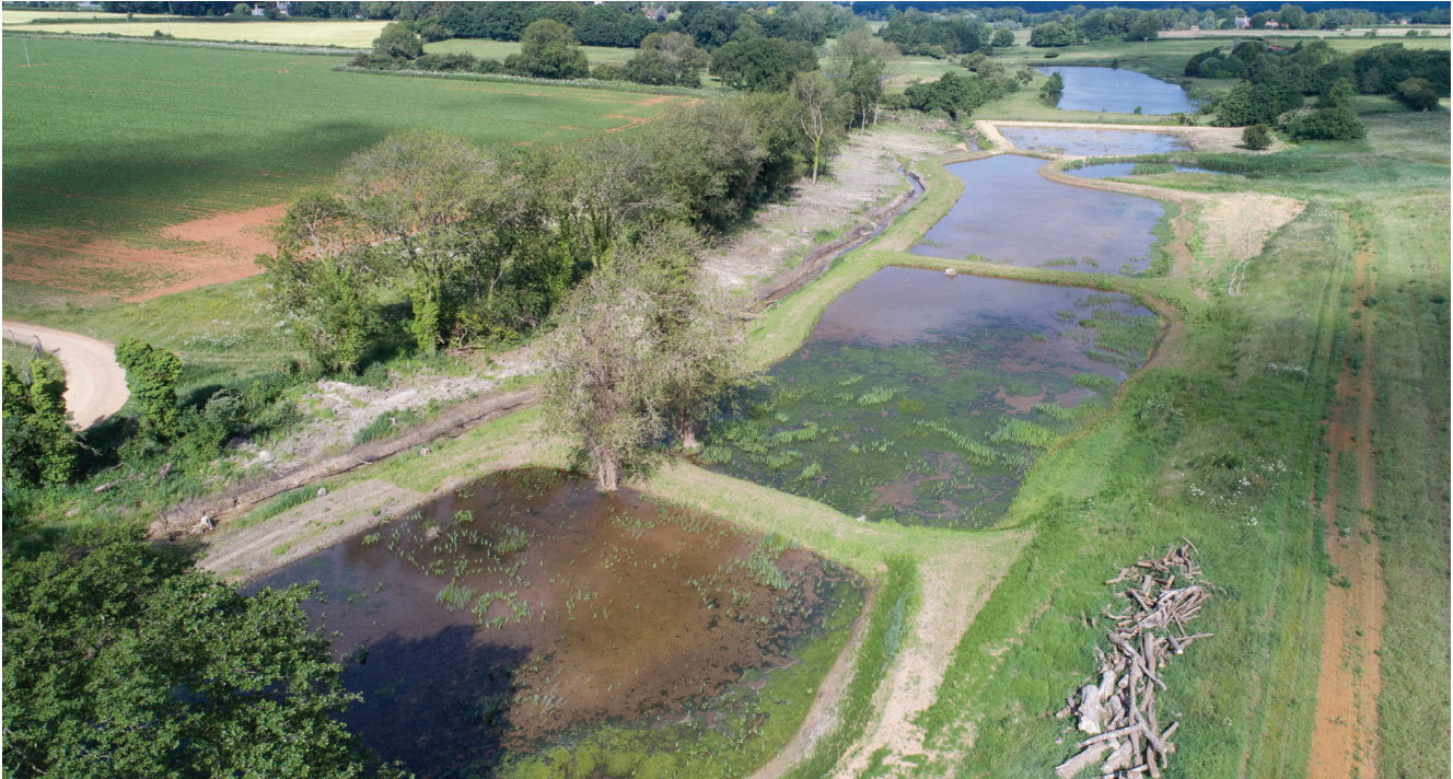
Aerial view of Ingodisthorpe recycling center with ponds forming the new treatment wetland © ANGLIAN WATER
