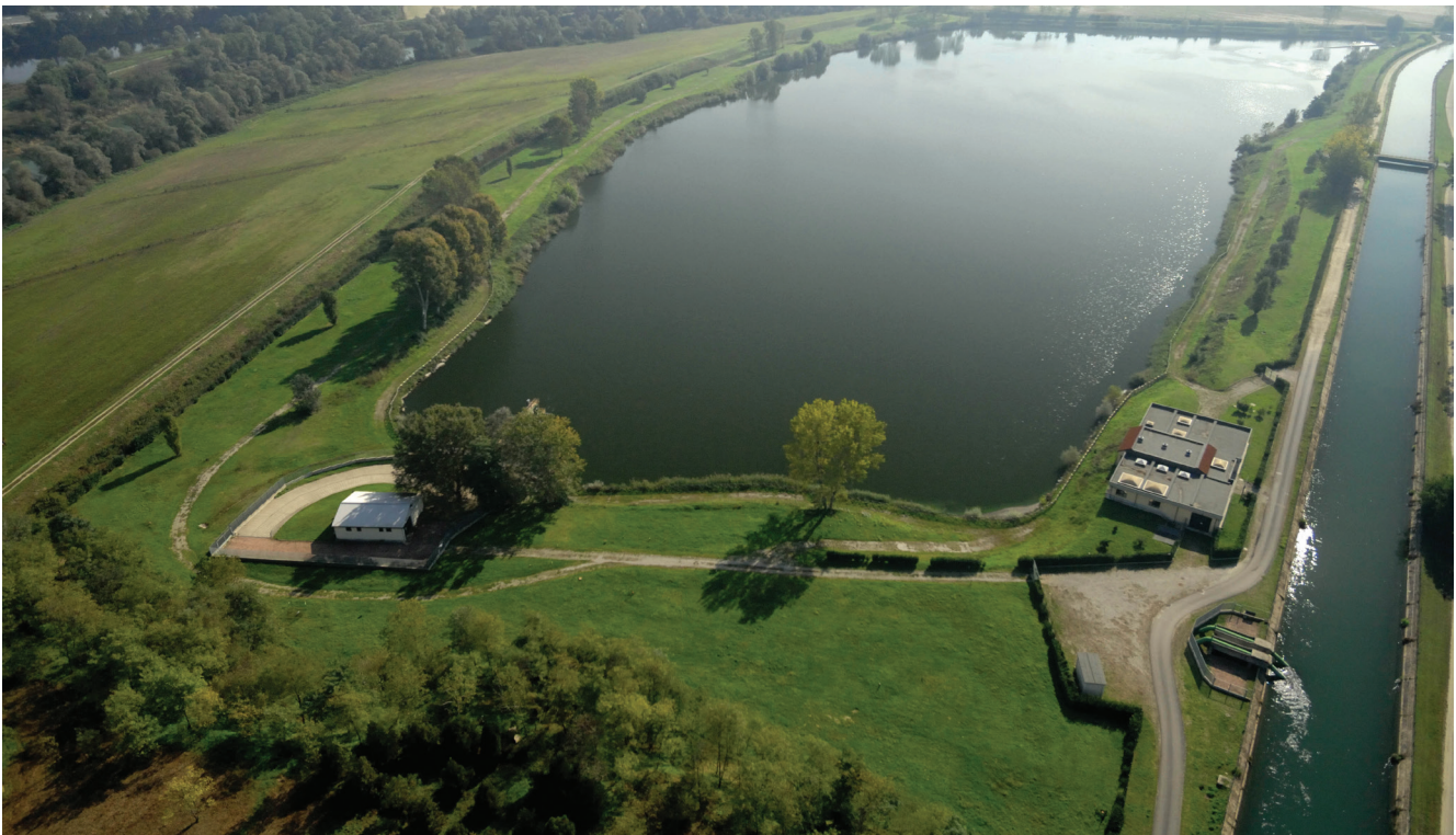
Aerial view of SMAT's raw water lagoon © SMAT
