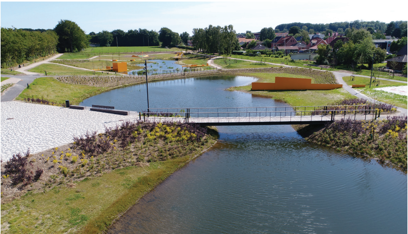
Rainwater lakes at Lasby Lake Park © SKANDERBORG FORSYNING
