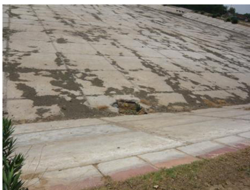
Figure 17.4 Hole in lining of facultative anaerobic pond.
