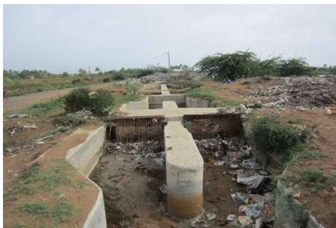
Figure 8.13 Poor maintenance of the primary treatment unit prior to WSP in the Municipal WWTP in City of Miraj, western India.
