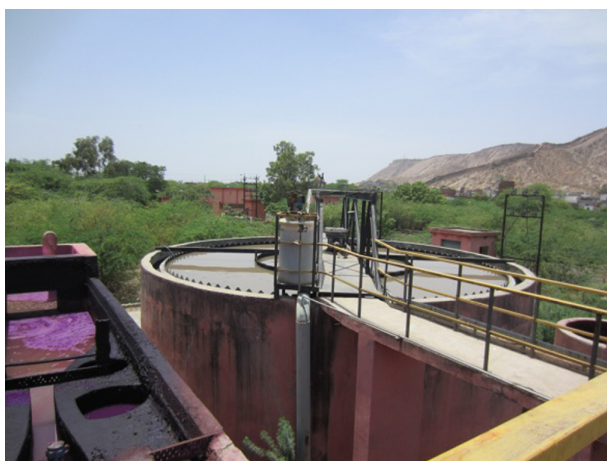
Figure 10.3 Removal of phosphorus using lime precipitation technology (first step in tertiary treatment).
