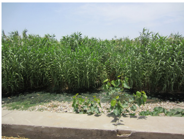
Figure 10.4 HSSF-CW (second step in tertiary treatment).
