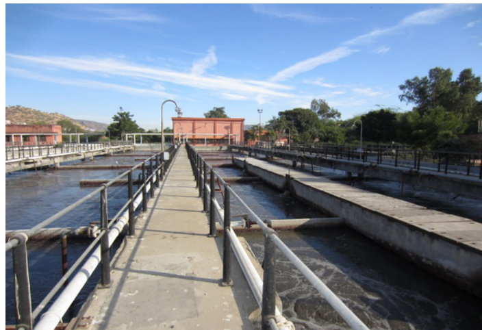
Figure 10.2 Conventional ASP to treat wastewater from the City of Jaipur ( \approx 27 MLD).
