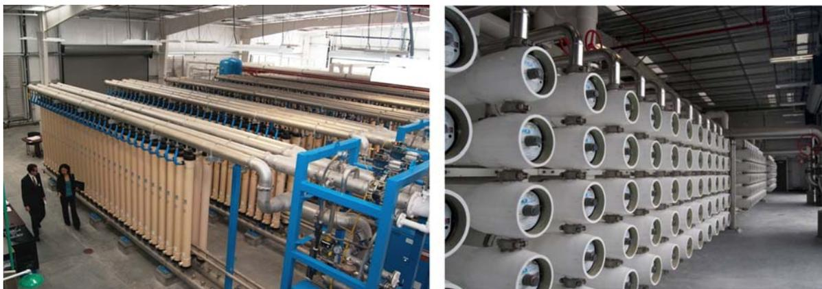
Figure 20.3 Views of the MF system and RO system.
