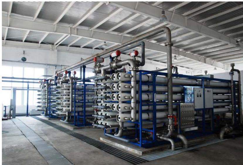
View of the reverse osmosis (RO) technology used to control recycled water salinity in Tianjin.
