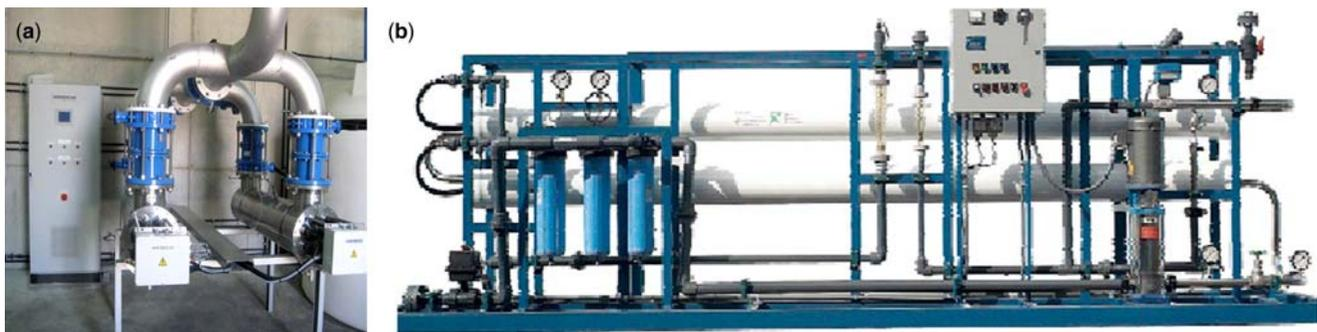
**Figure 8.3** Views of UV disinfection (a) and ultrafiltration modules (b).
