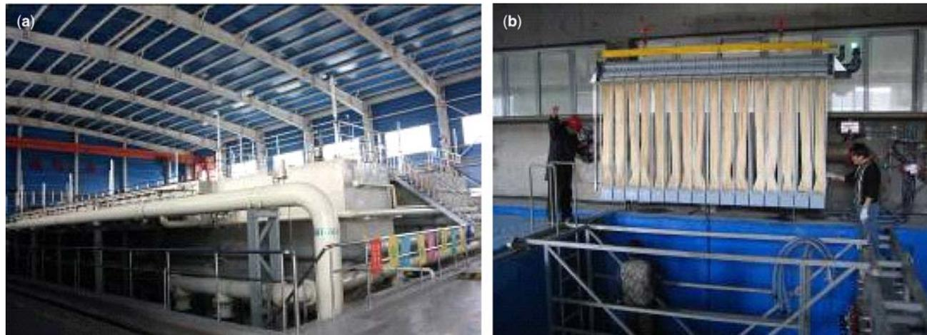
**Figure 23.4** Views of the QingHe water reclamation plant (a) and the BeiXiaoHe water reclamation plant (b). (a) Tertiary filtration – ZeeWeed 1000 membrane tanks (b) MBR – installation of a Memcor Memjet module.
