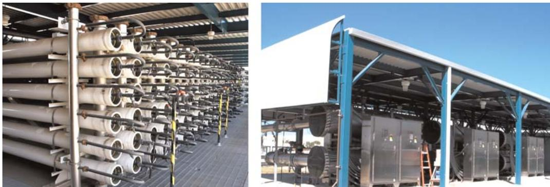
Figure 2.2 View of reverse osmosis and the advanced oxidation by UV/H<sub>2</sub>O<sub>2</sub>.
