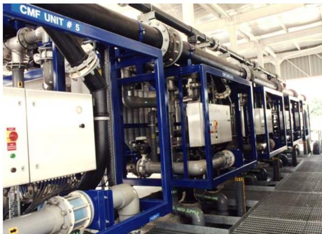
Figure 3.4 NEWater production process: view of microfiltration.
