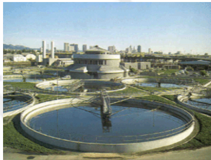
Clarifier at the Main Wastewater Treatment Plant in Oakland
