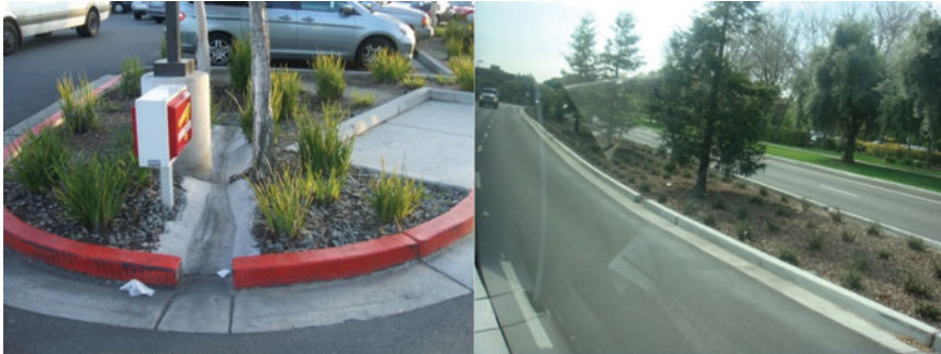
Figure 12.1 Bad design: flow channels were not properly designed so runoff cannot be diverted into the facilities for infiltration (San Francisco/California).
