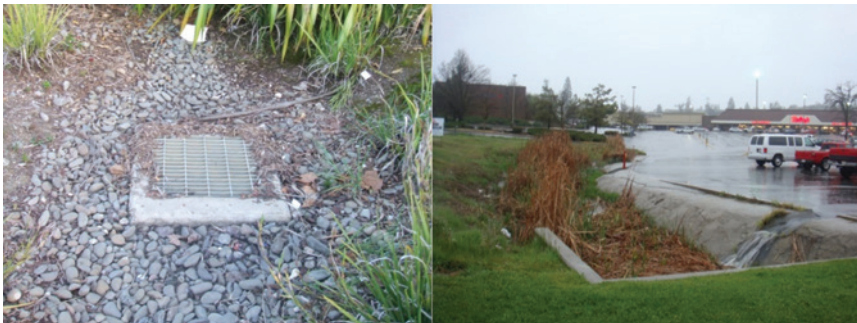
Figure 12.2 Bad management: overflow pipe in bioretention ( above left ) and small constructed wetland ( above right ) blocked with litters (San Francisco/California).
