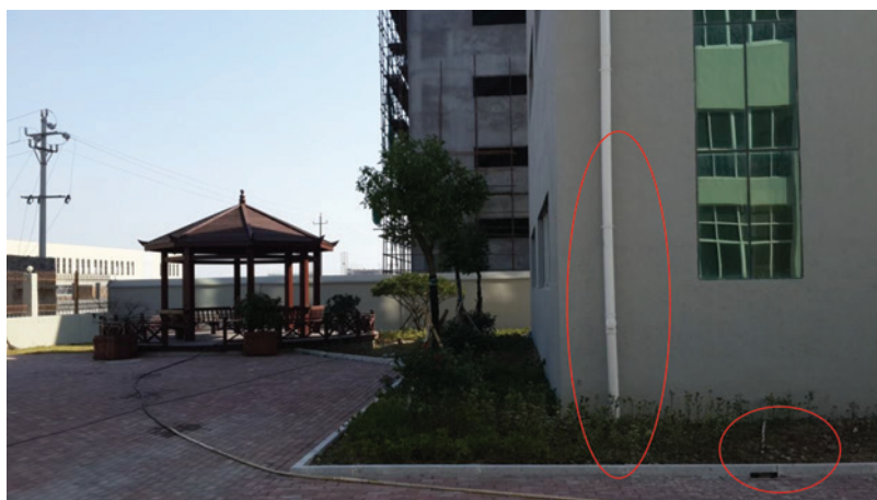
Figure 8.5 Disconnection of roof downspout and rain garden.
