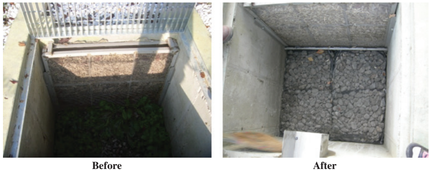
Figure 12.13 Filter media were packed for ease of maintenance in the infiltration trench as part of the non-routine maintenance.
