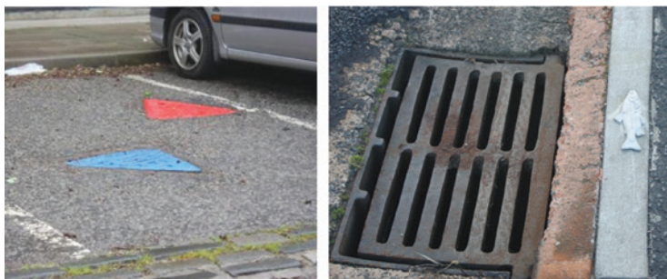
Figure 17.16 Trying to prevent pollution from misconnections or casual disposal into the wrong drain.
