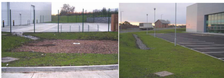
Figure 4.4 Examples of SUDS at industrial estates.
