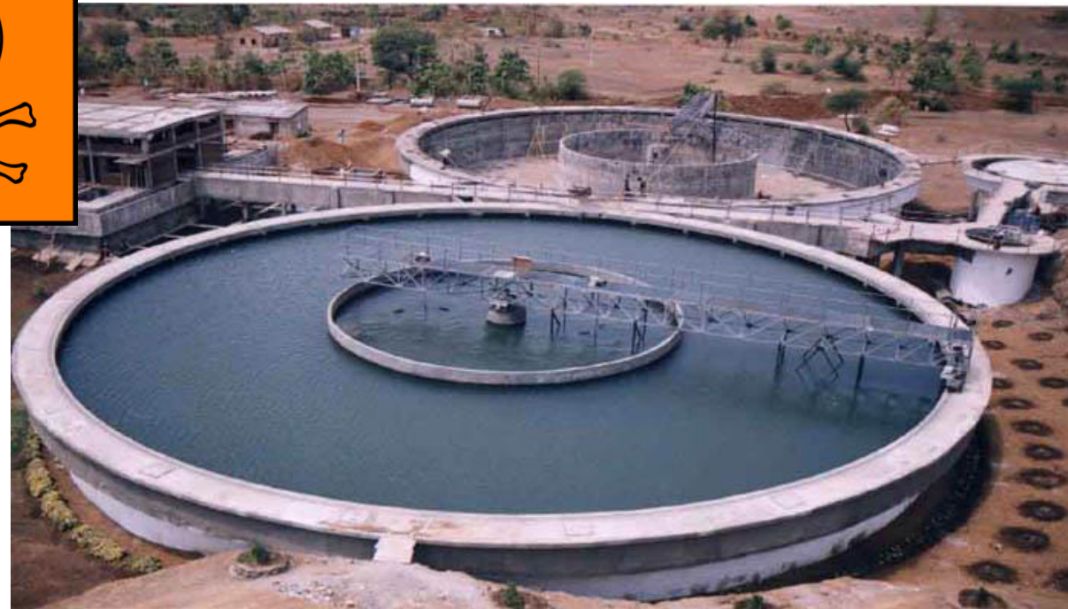
Large flocculation tank in operation
