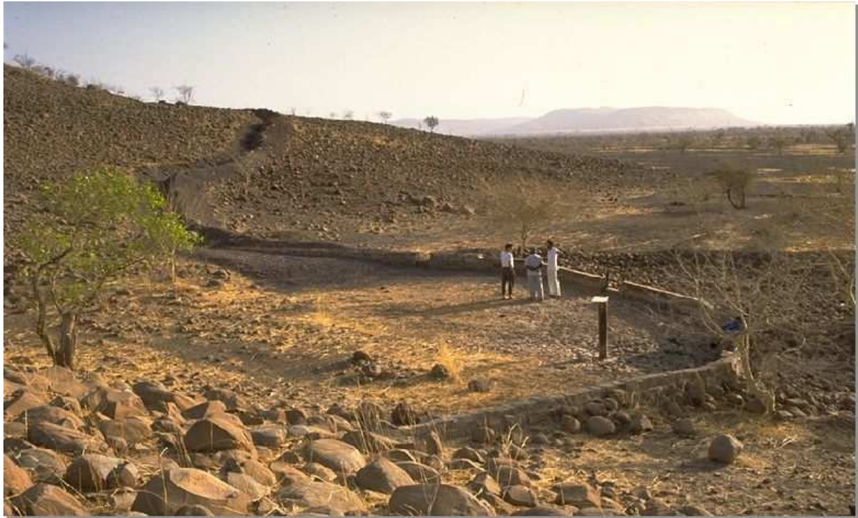
Figure 10: Example of macro-catchment water harvesting (hillside conduit, photo: Klemm)
