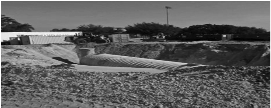
Figure 9.4 Patel Centre cistern installation.
