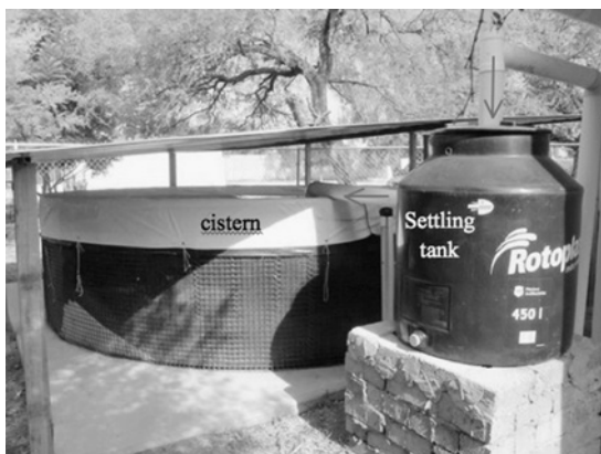
Figure 6.2 Typical above-ground cistern/storage and settling/sedimentation tank.
