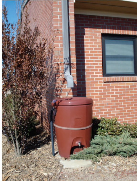
Figure 2.8. Rain Barrel at Fort Bragg
