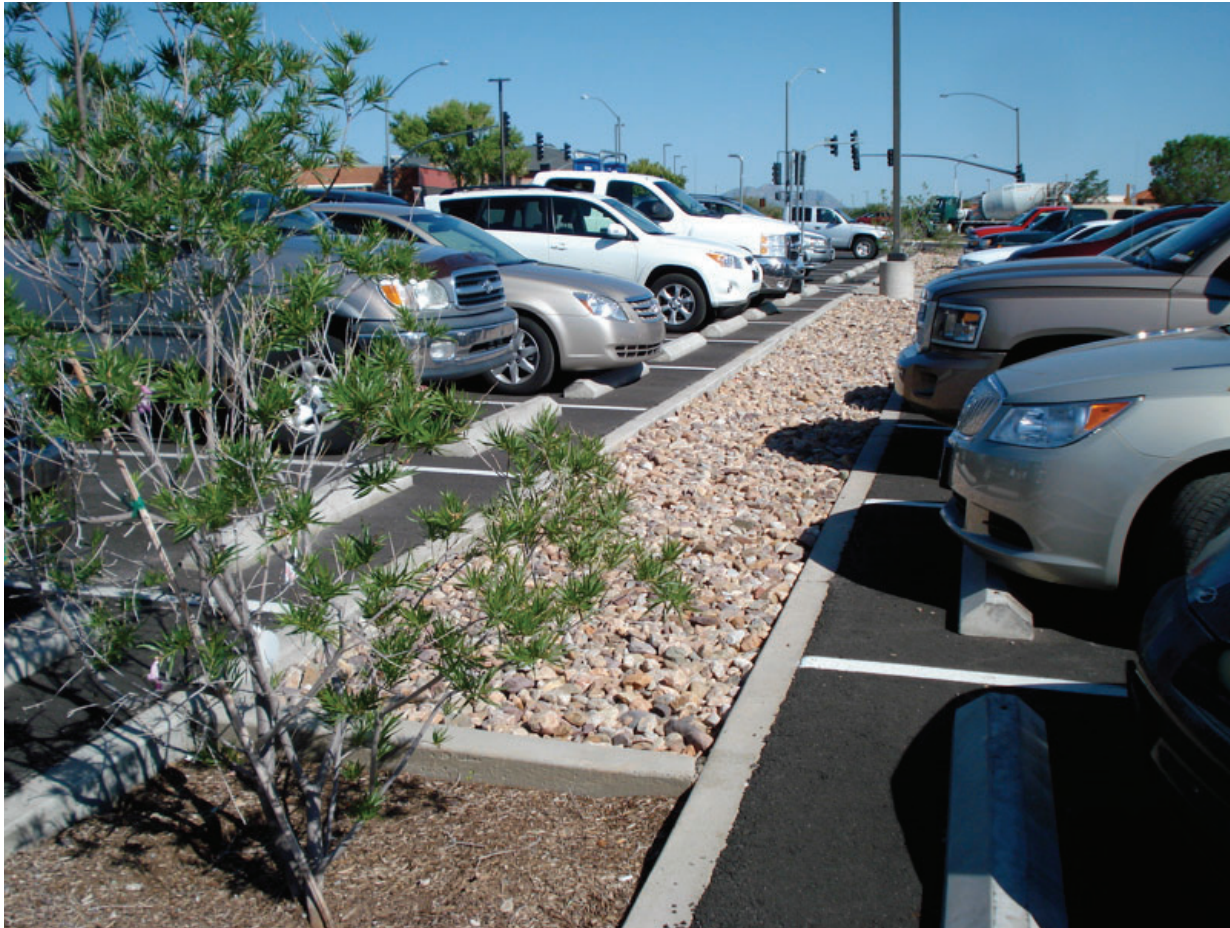
Figure 6.14. Fort Huachuca Commissary Parking Lot Area Designed to Better Manage Stormwater Runoff
