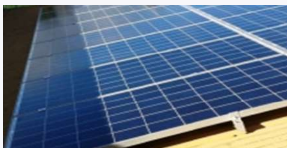
Figure 49: Building gets constructed near your mounting structure
