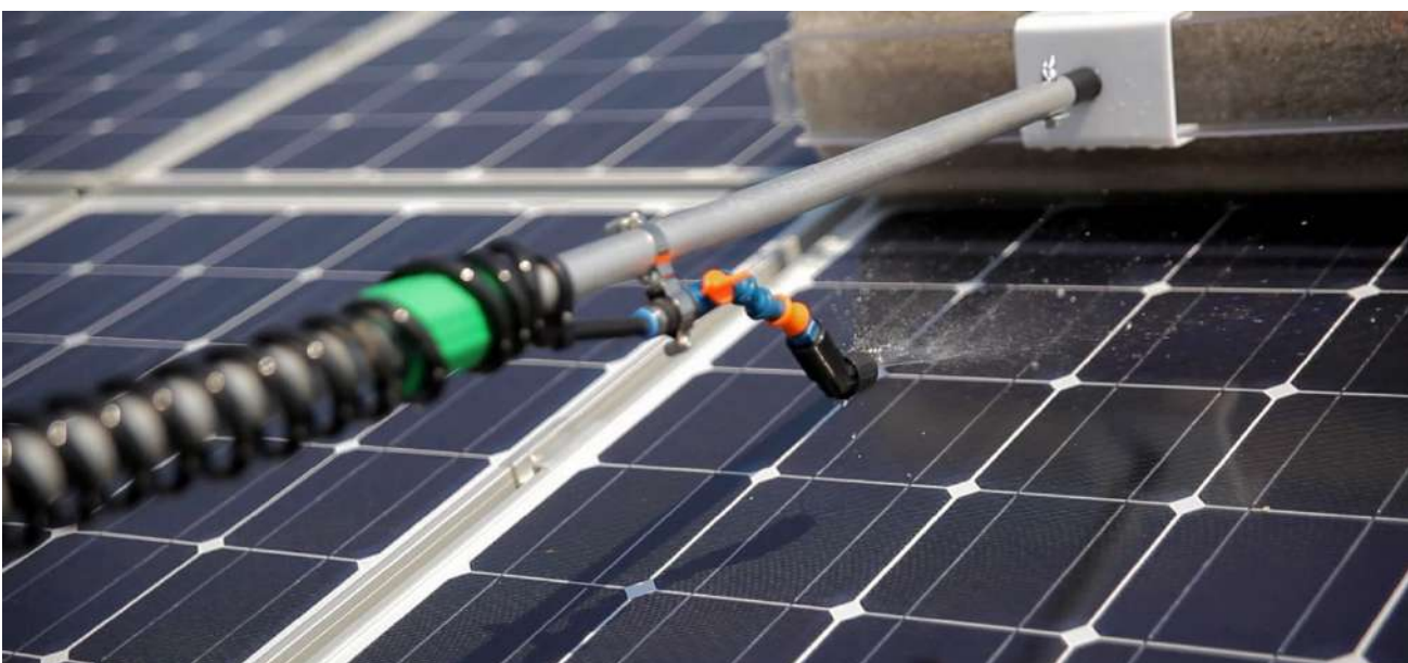
Figure 45: Wet cleaning using an automated system
