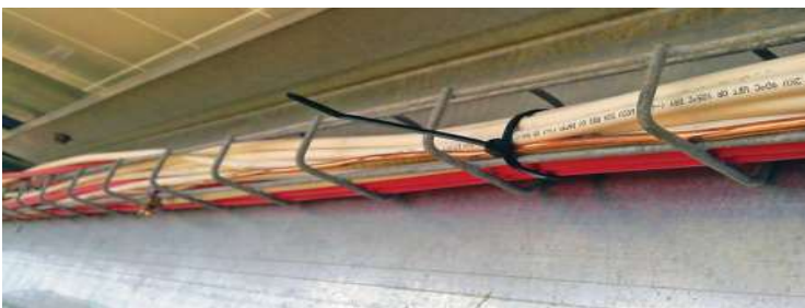
Figure 113: Cables are tied using cable tie
