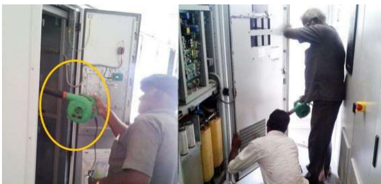
Figure 89: Cleaning inverter using blower
