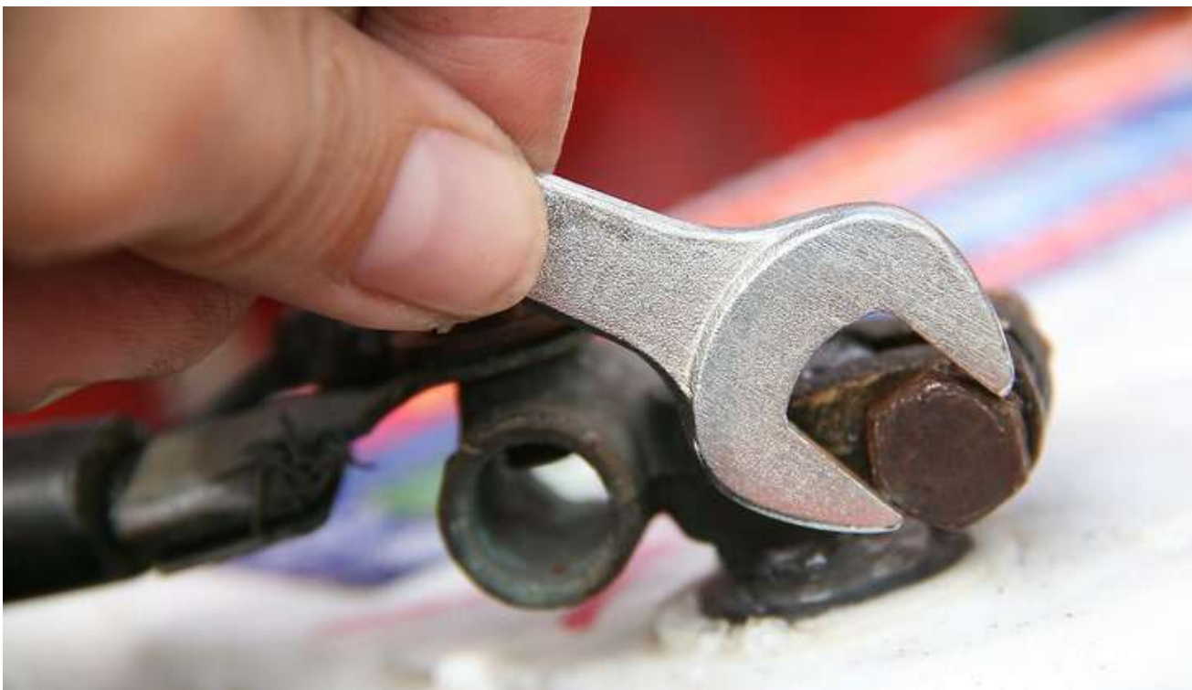
Figure 131: Tightened battery terminals
