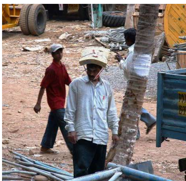
Figure 150: Incorrect practice - Without safety helmet
