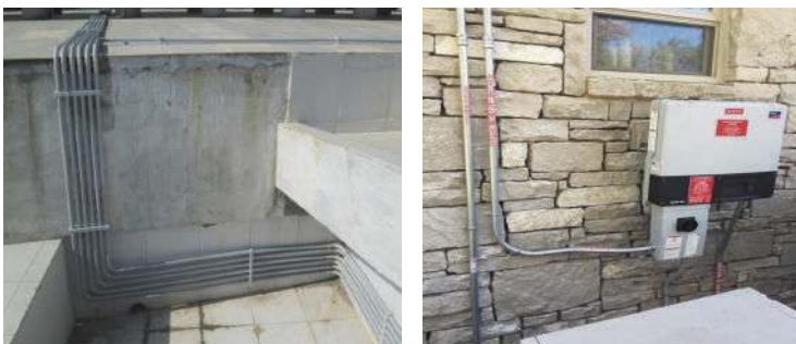
Figure 101: Proper cable routing
