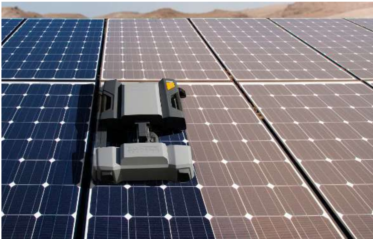
Figure 46: Dry cleaning method using an automated system
