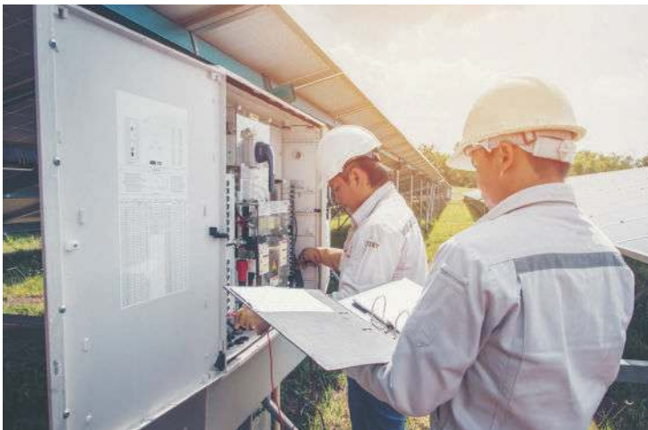
Figure 94: Written inspection report of Inverter
