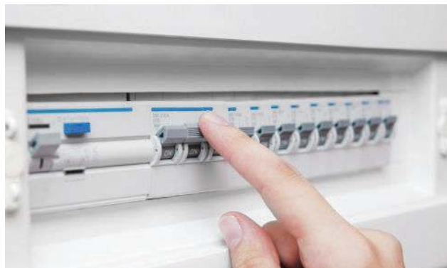
Figure 74: Switch off inverter before performing any maintenance
