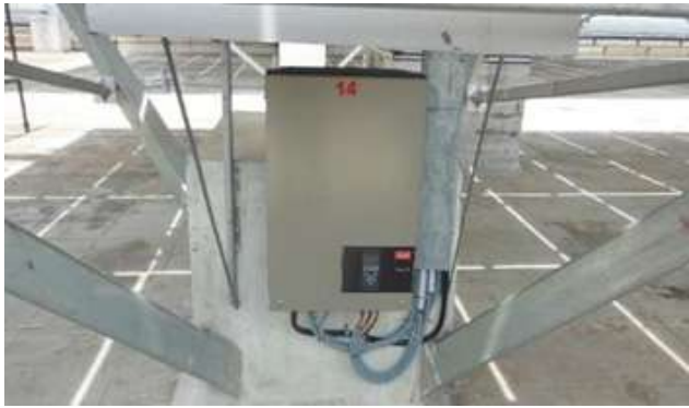
Figure 93: Inverter grounding levels
