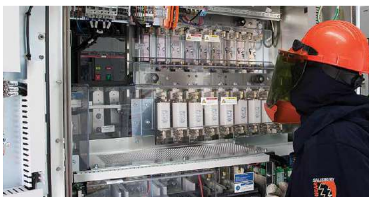
Figure 92: Check inverter fuses
