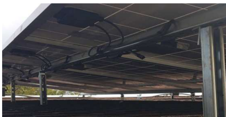
Figure 104: Correct cabling connection
