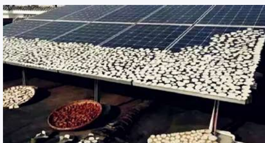
Figure 50: Shading due to drying crops
