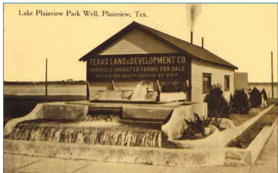
FIGURE 41. Park well for the Texas Land & Development Co. office in Plainview, Texas (circa 1910).
