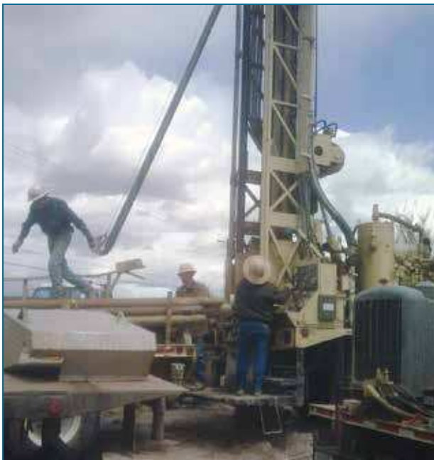
FIGURE 37. Drilling and installing a well. (Source: Gary Hix)
