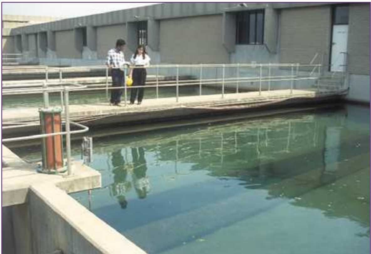
Figure 12: Photograph of rapid gravity sand filter
