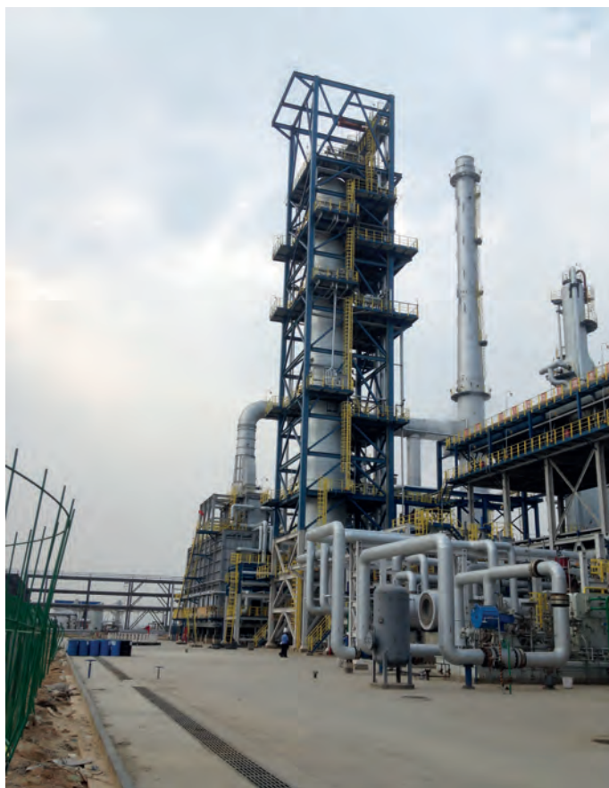
Figure 1. An IsoTherming reactor in commercial service.
