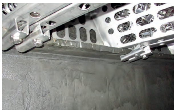
Figure 3. The 2021 inspection of HVTS applied by IGS in 2015 shows the cladding in excellent condition.
