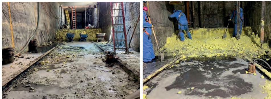
Figure 3. View of sulfur cake and carsul removal from a four-year decommissioned sulfur pit that was recommissioned and brought back online at a Midwest US refinery.
