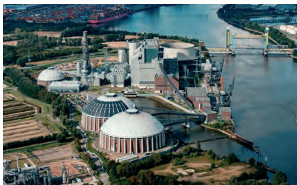
Figure 1. At Moorburg, a mega-electrolyser will be the heart of the HGHH. Source: Mediaserver Hamburg/Doublevision.
