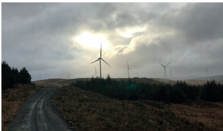
Figure 1. Mercury is developing one of Ireland's first co-located onshore wind farm and hydrogen electrolysis plants.
