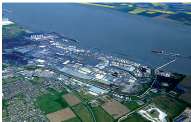
Figure 1. Aerial view of ABP's Port of Immingham.
