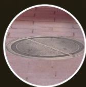
Sewer Forcemain Discharge
