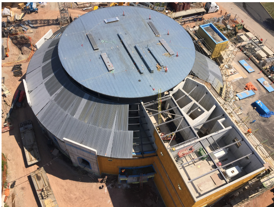
The new raw sewage pumping station at Woodward Avenue. Courtesy of Reimar Construction
