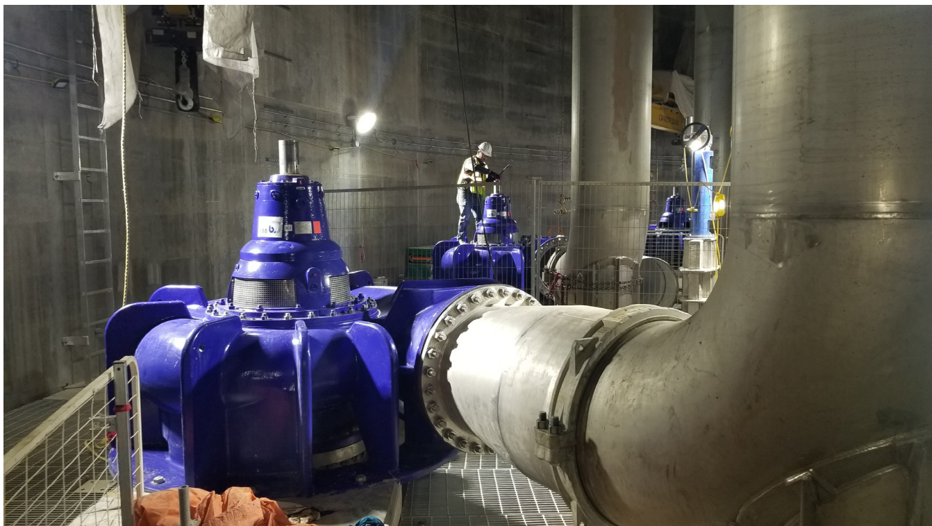
The first of the pumps being installed and anchored to their mountings. Courtesy of KSB Canada.
