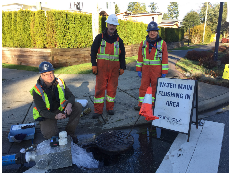
Operators of the water department working on one section of the unidirectional flushing program. City of White Rock
