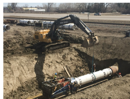
Phase 2A of the Malloy Drain implementation project in the Town of Coaldale, Alberta, cost $5.4 million. Alberta Irrigation Districts Association
