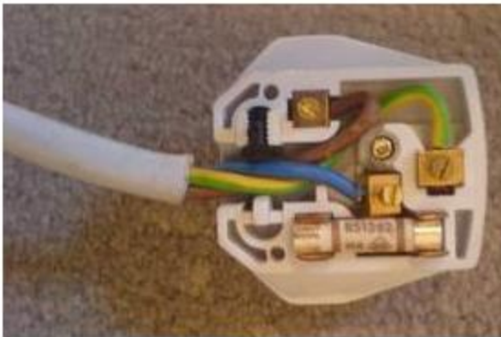
Outer cable insulation not secured into the plugs
