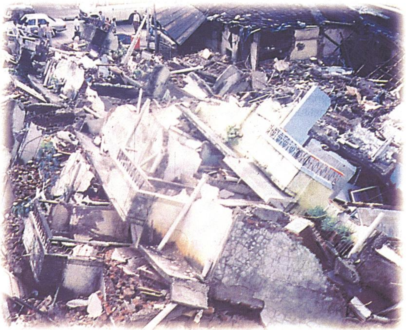
Figure 12 : Those whom God love die young. "Shiv Chandan" building barely a teenager collapsed at Amboli Naka, Andheri, Mumbai on 1st September 1994.
