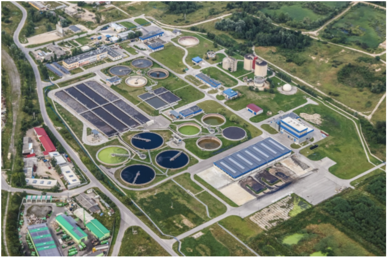
Wastewater Treatment Plant: Photo by Michal Jarmoluk on Pixabay.
