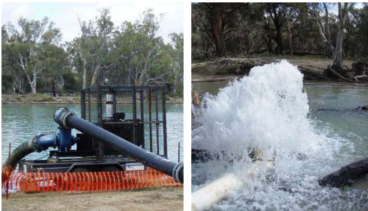
Figure 11. Water being pumped by the Murray Wetlands Working Group into a wetland near Mildura. Photos L. Beesley.
