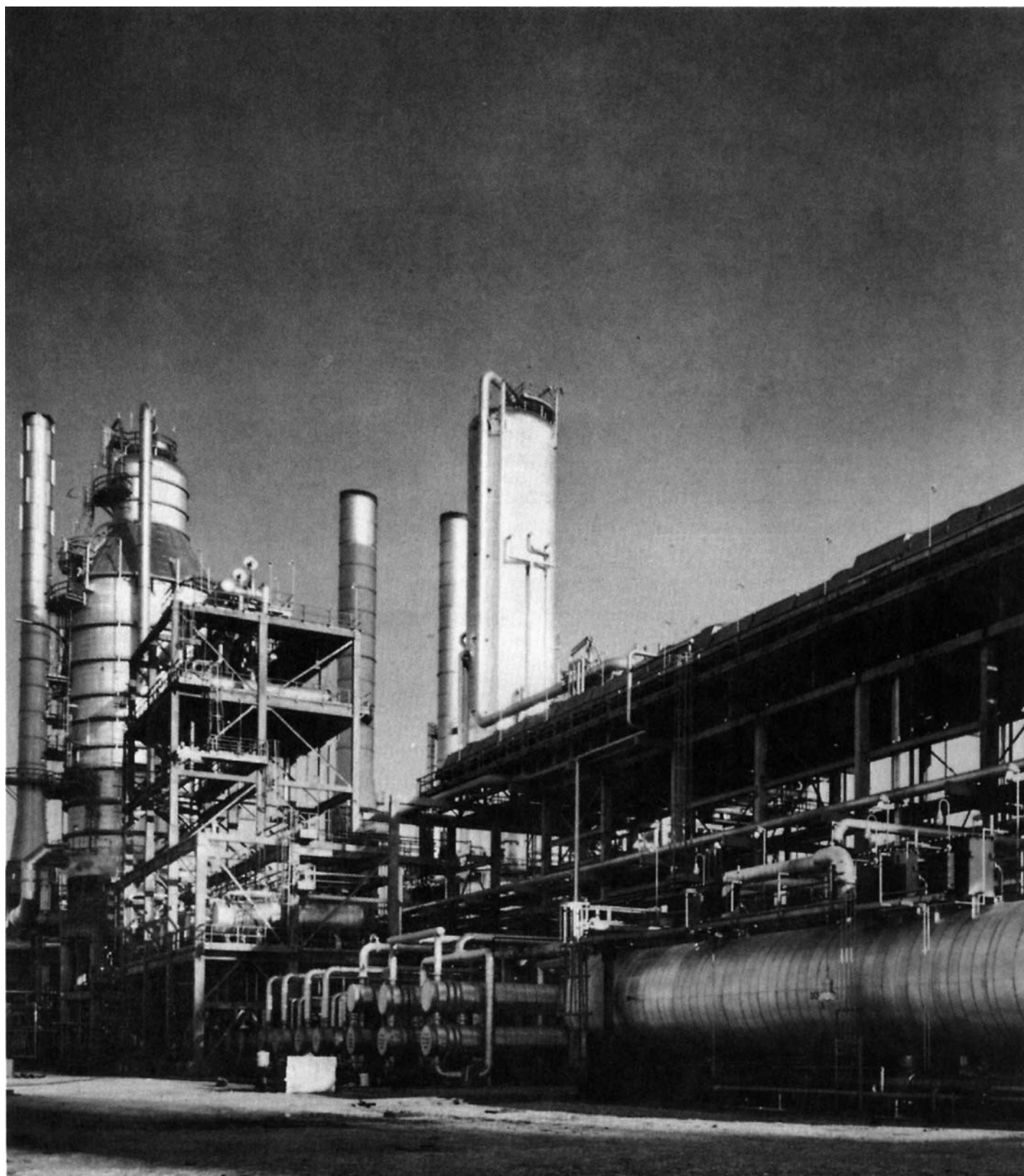
Crude unit desalters at the Marathon Oil Company Garyville Refinery. The crude vacuum tower is shown at the left.
