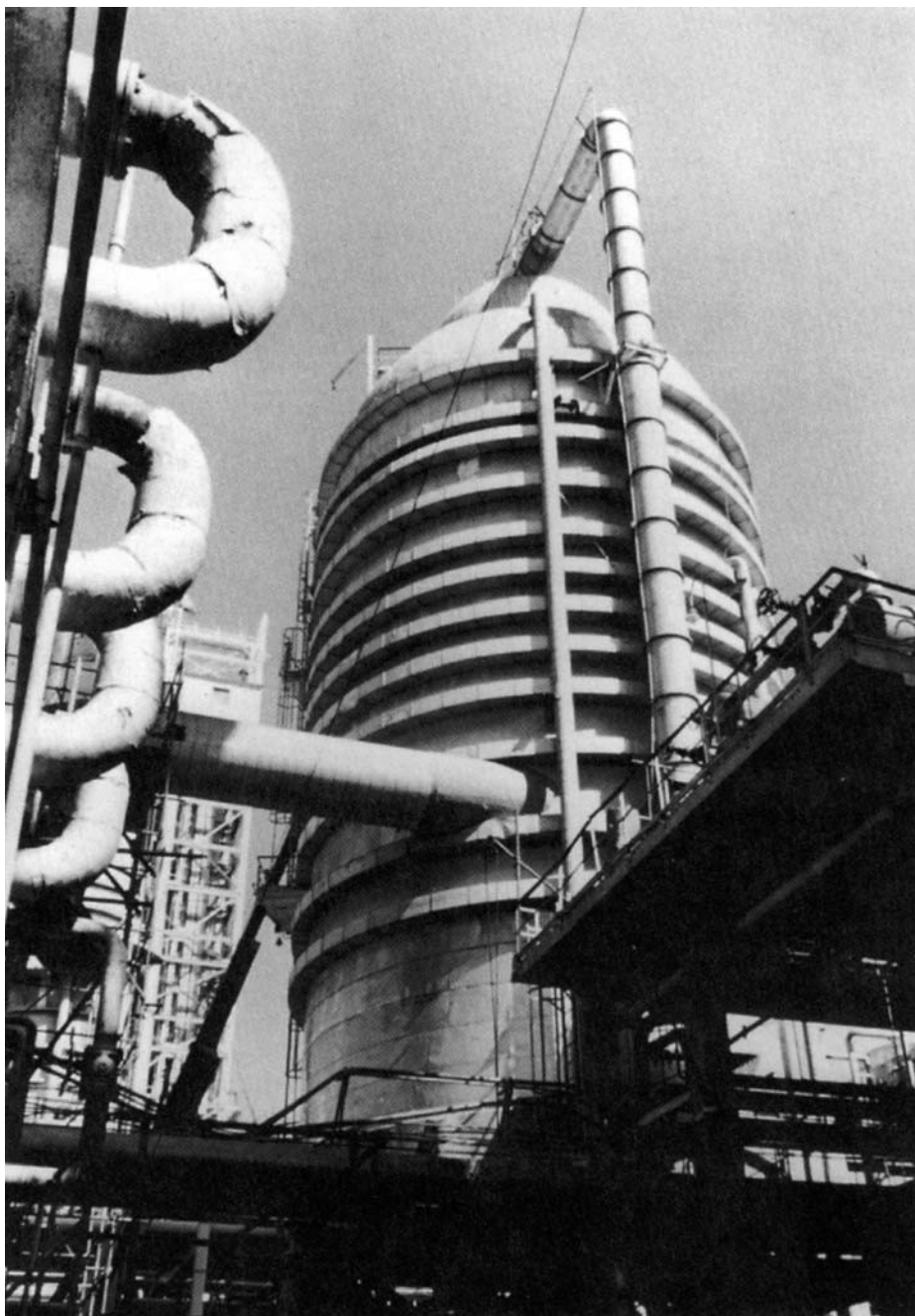
Vacuum distillation tower has Type 316 stainless steel lining and trays for protection against corrosion by naphthenic acid. Cross-over elbows (left foreground) are also Type 316.
