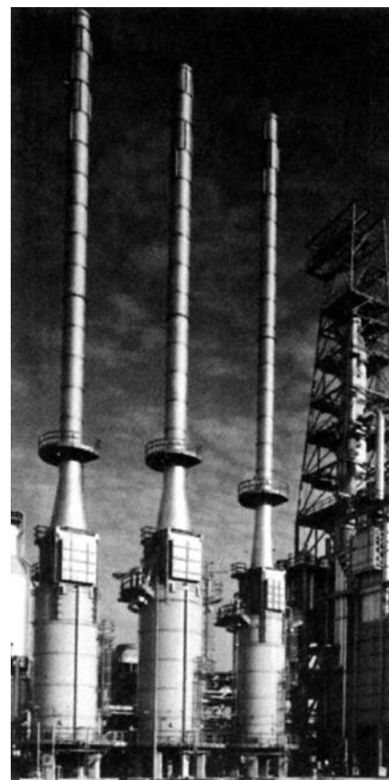
Catalytic reformer section of Marathon Oil Company Garyville Refinery showing Platformer fired heaters.
