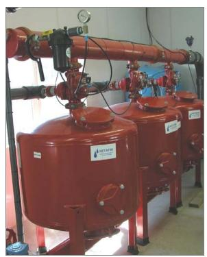
Figure 3.3. A sand filtration system in the pumphouse.
