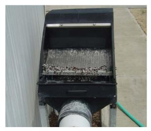
Figure 1.2. An example of a coarse filter in a greenhouse irrigation system. A finer filtration system would improve the efficacy of ultraviolet light and other treatment systems.
