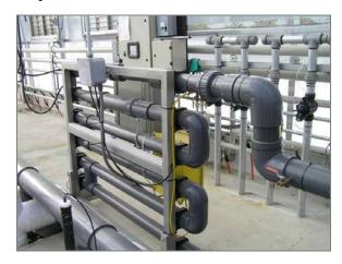
Figure 9.3. Installation of a copper ionization system in a commercial greenhouse operation.
