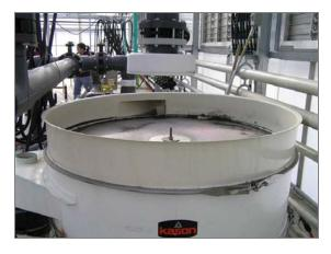
Figure 9.2. A copper ionization system can be combined with other water treatment technologies such as filtration.
