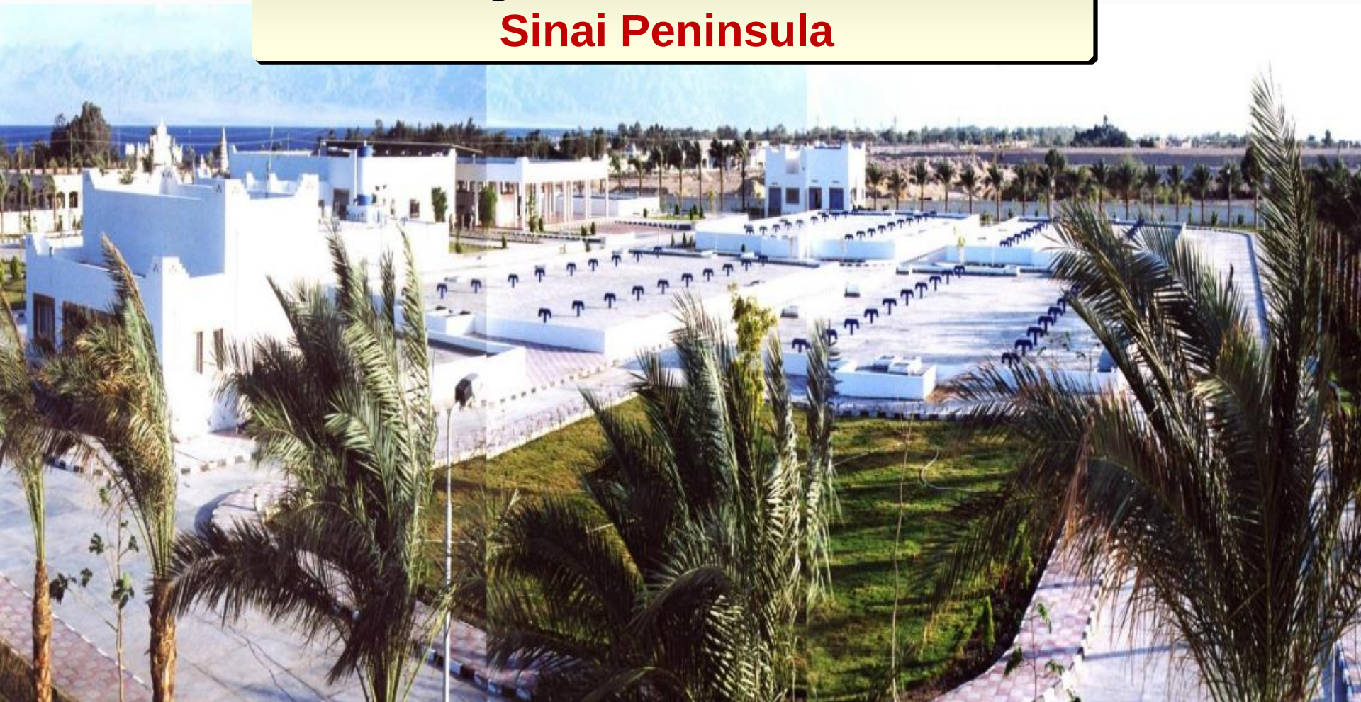
Nuweiba Desalination plant ( 10000 m 3 /day )
