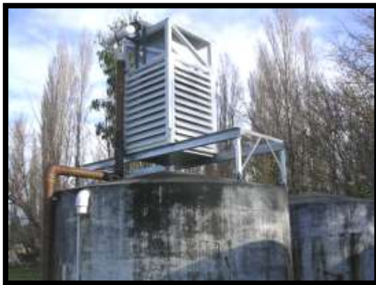
Figure 8: Simple aeration unit
