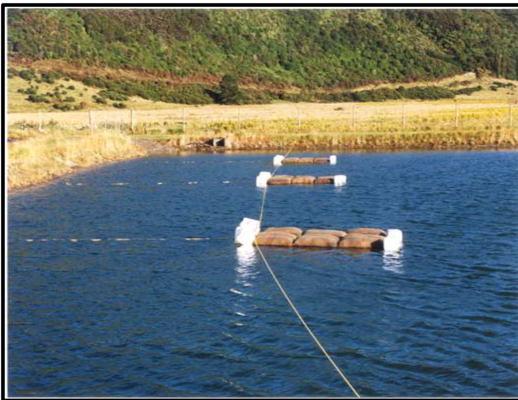
Figure 3: Raw water reservoir
